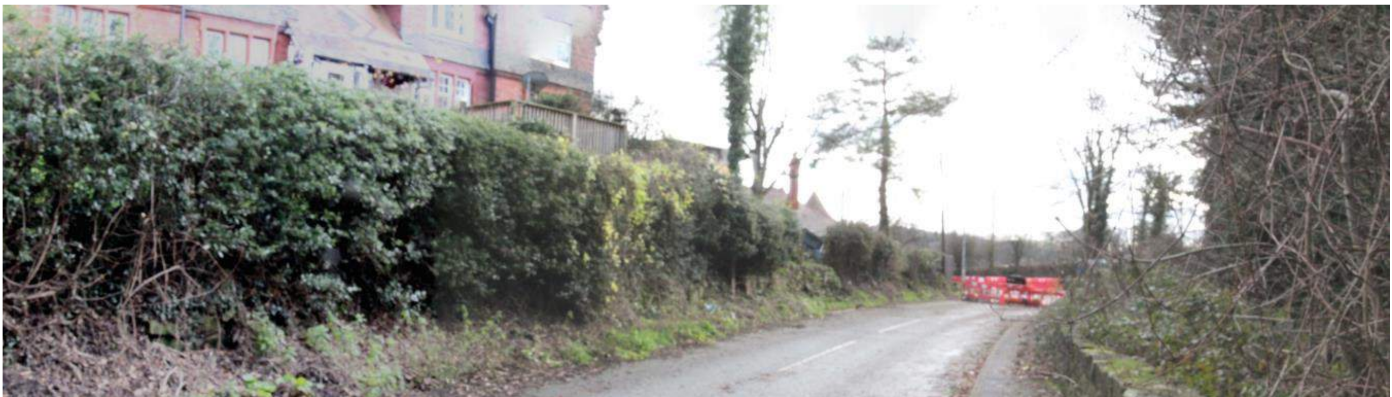
Plate 6 — Photograph taken from the pavement of the B5605 (Currently closed to vehicular traffic due to a landslip) approaching the proposed site from the northerly direction of Cefn Mawr
