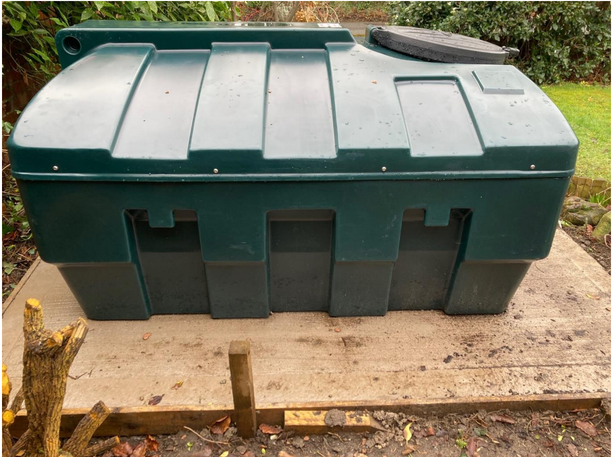
Left side elevation of tank in situ
