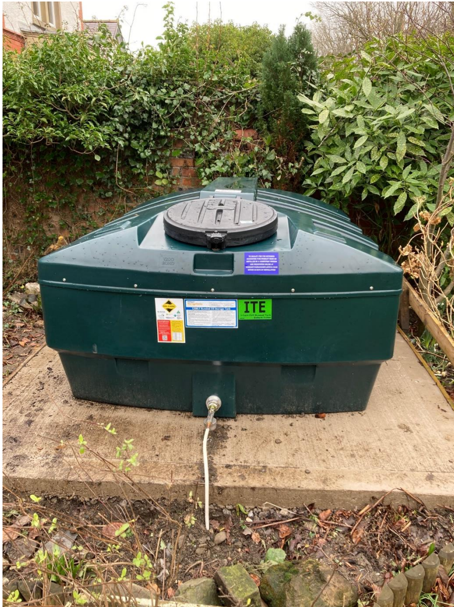
Front elevation of tank in-situ
