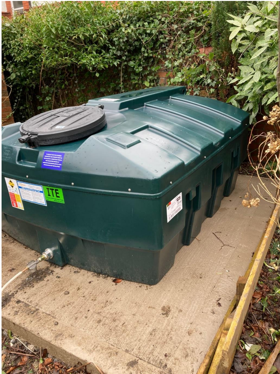
Right side elevation of tank in-situ
