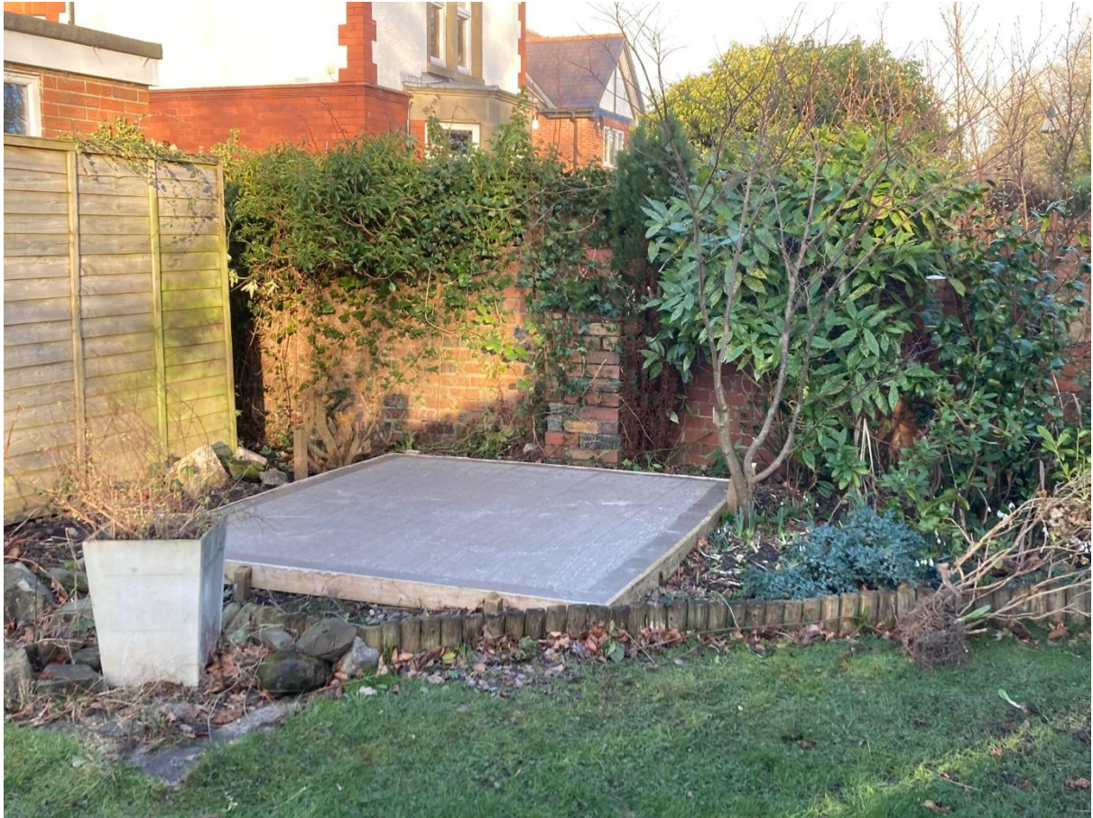
Base for replacement tank for domestic heating oil in-situ
