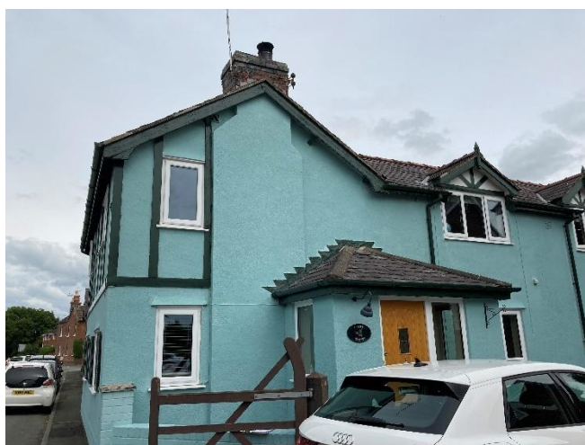
Figure 2 – Image taken on Architect's Survey.
