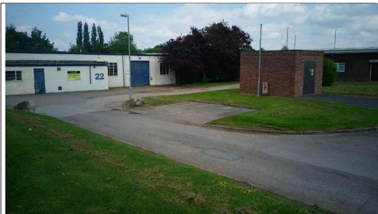
Plate 13: On site sub station
