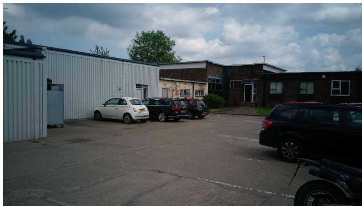
Plate 2: The Bridgeway Centre
