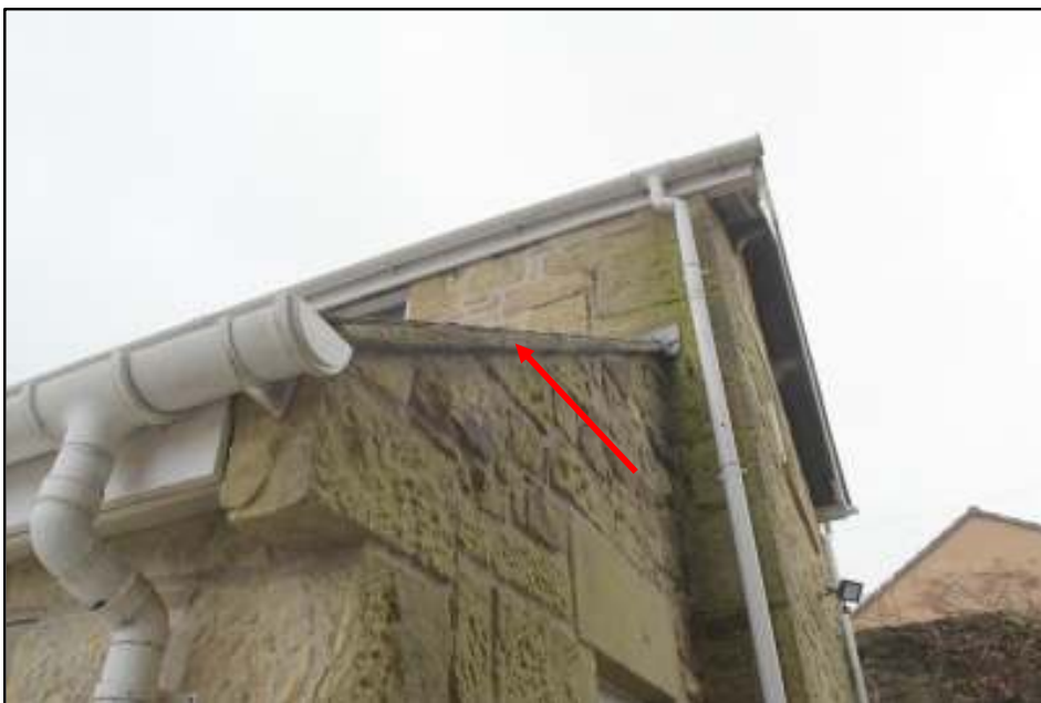
Side section of the garage is well sealed below the slate edge
