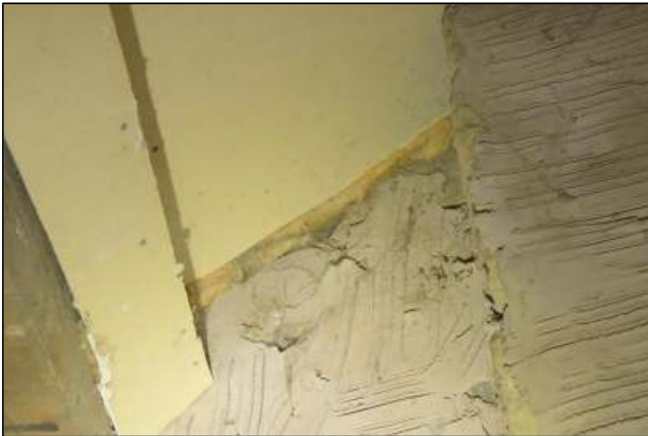
Insulation under the plaster board fills the cavity
