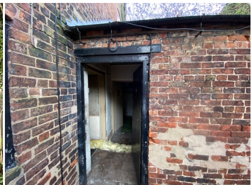
Rear side of kitchen annex and kitchen doorway with damaged brick adjacent
