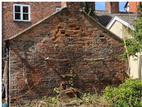
Rear side of kitchen annex and kitchen doorway with damaged brick adjacent
