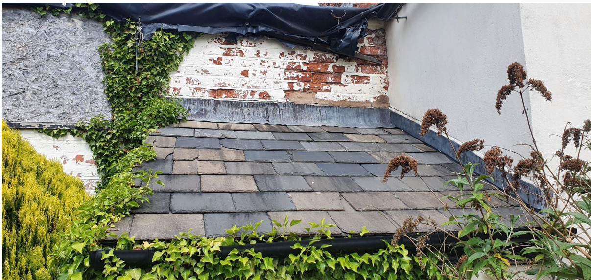
Plate 6: An image of some of the lifted lead flashing on the structure.
