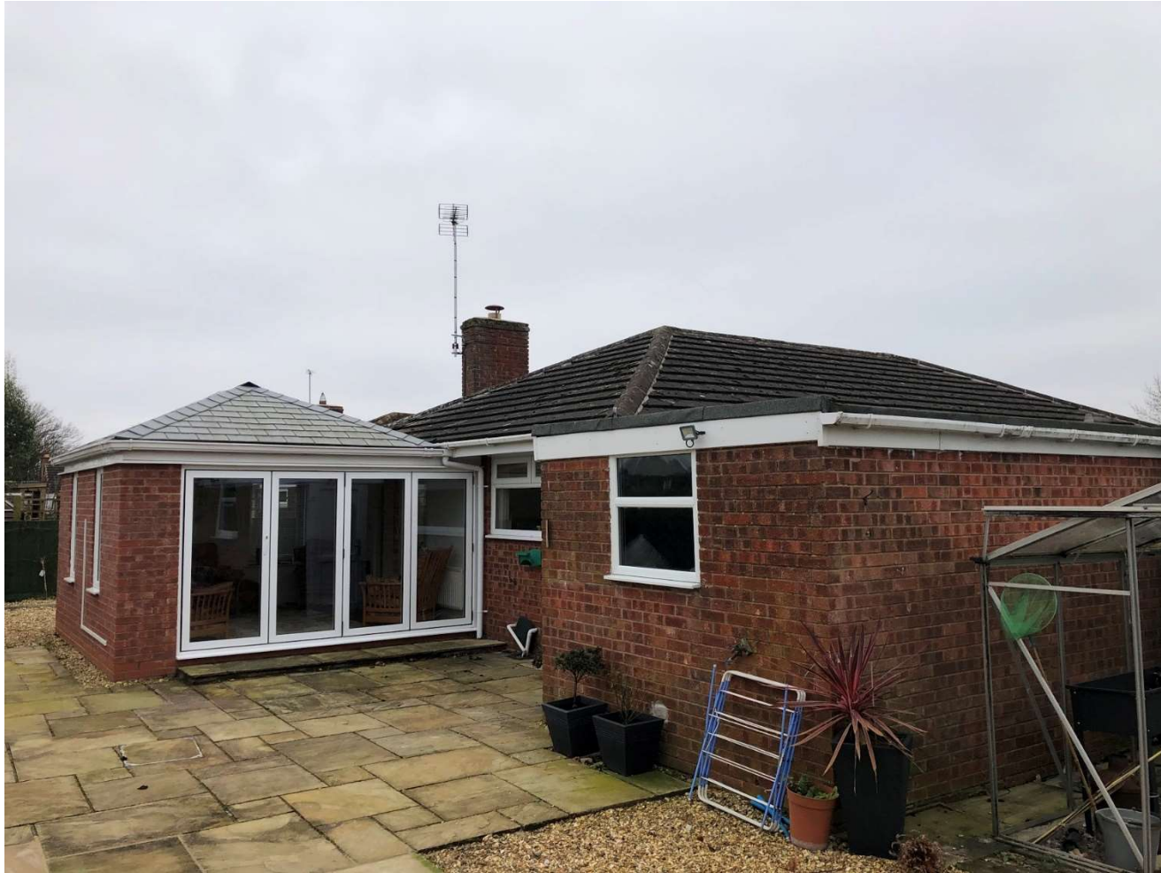
View Southwards towards rear of property
