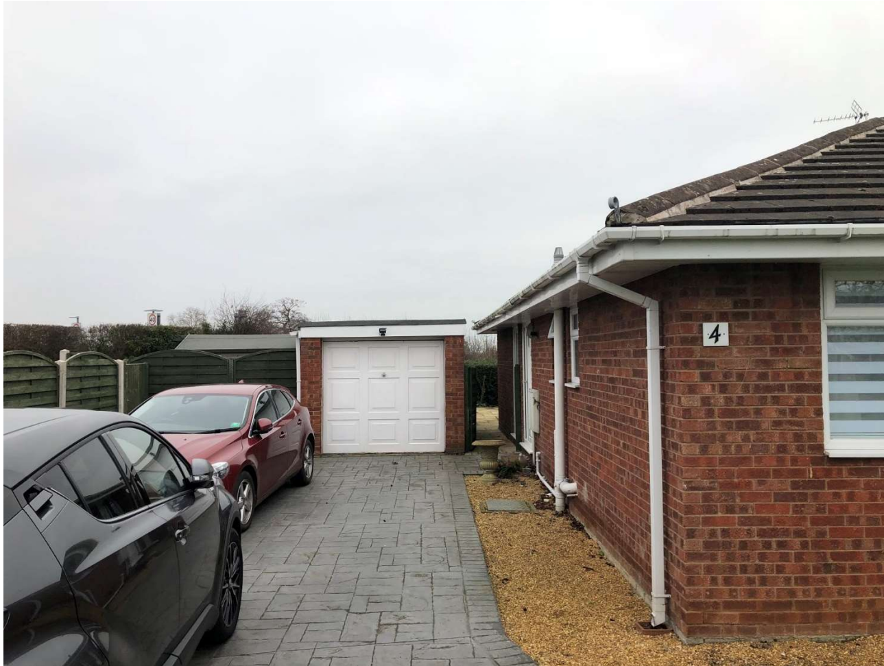
Existing front elevation (view from Driveway towards location of proposed extension)
