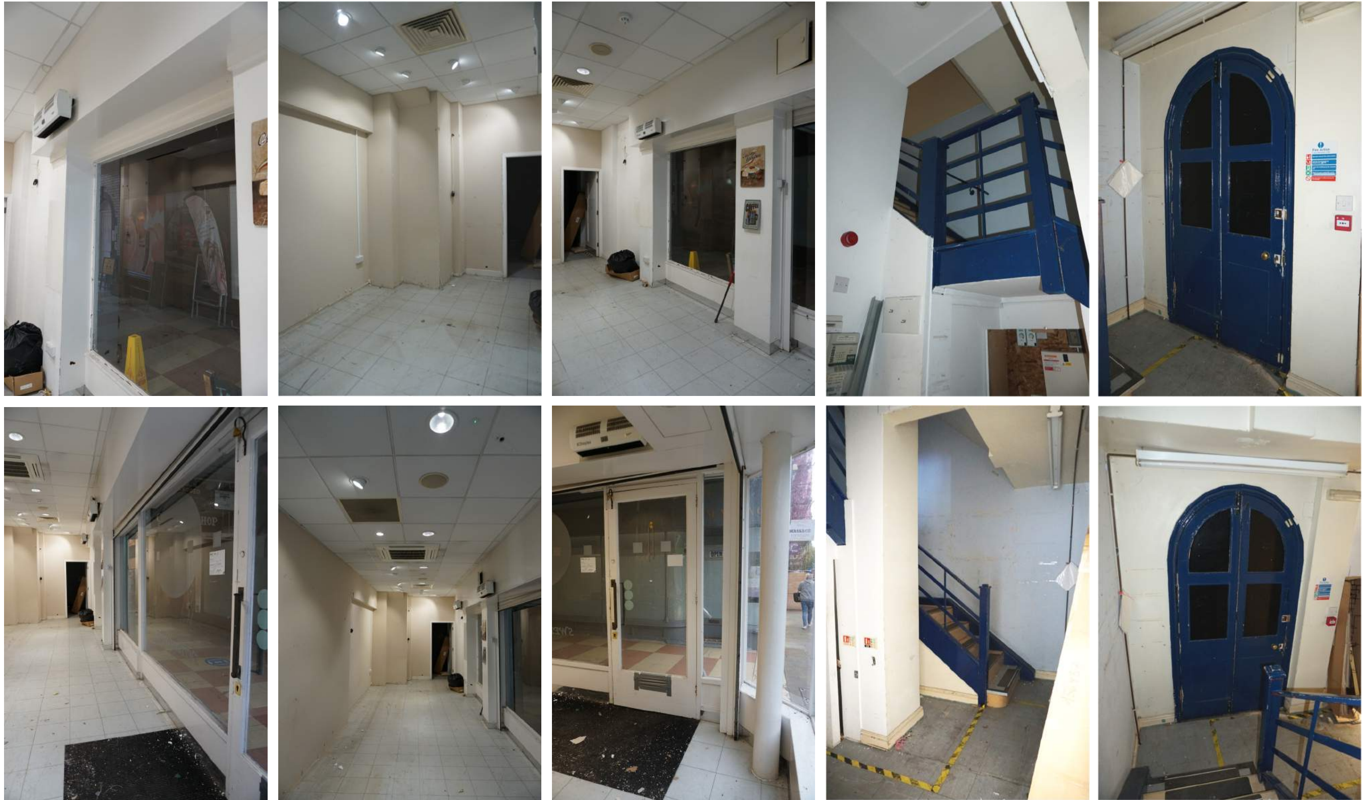
EXISTING GROUND FLOOR PHOTOGRAPHS
