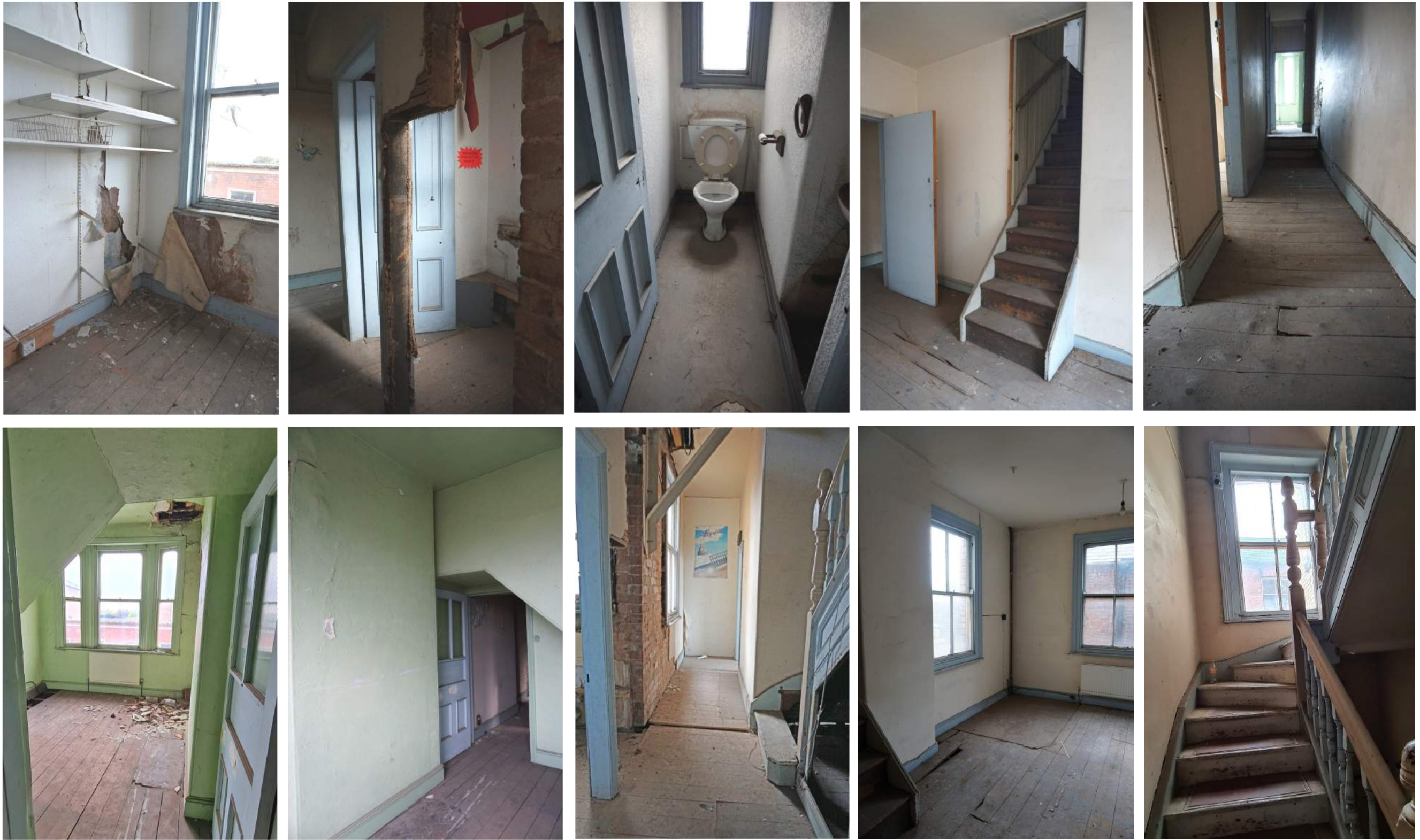
EXISTING SECOND FLOOR PHOTOGRAPHS
