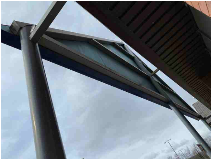
5 MAIN SIGN - REAR EXISTING
