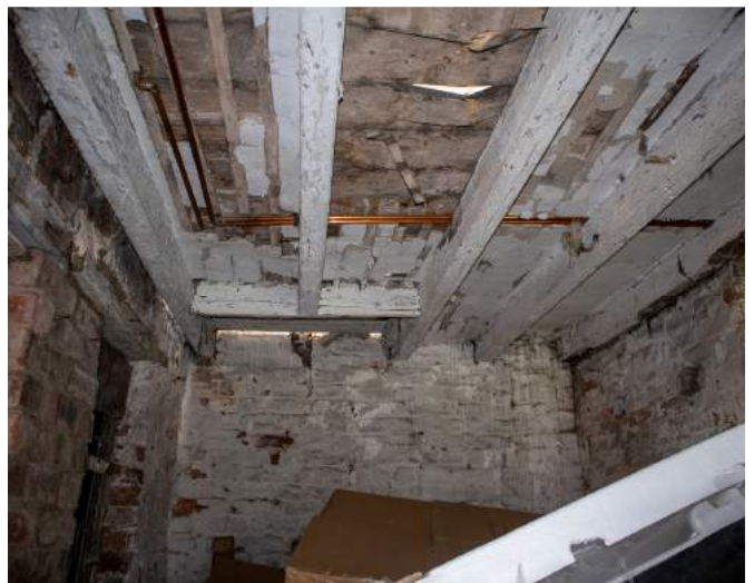
Photograph B4: (6749) Internal view of the first floor joists over the garage. Generally, the joists were in a satisfactory condition.
