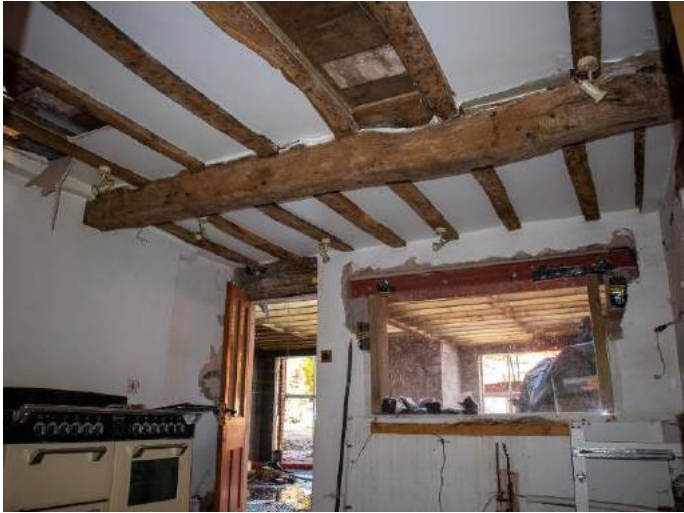
Photograph B1: (6734) View on the ceiling structure to the kitchen.
