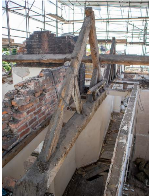
Photograph B6: (6772) View on truss 2 with Truss 1 in the distance. Note that the condition of the timber is generally satisfactory; the landing wall is solid bonded masonry and supports the overlapping purlins; the bathroom wall is stud construction running parallel with the truss.
