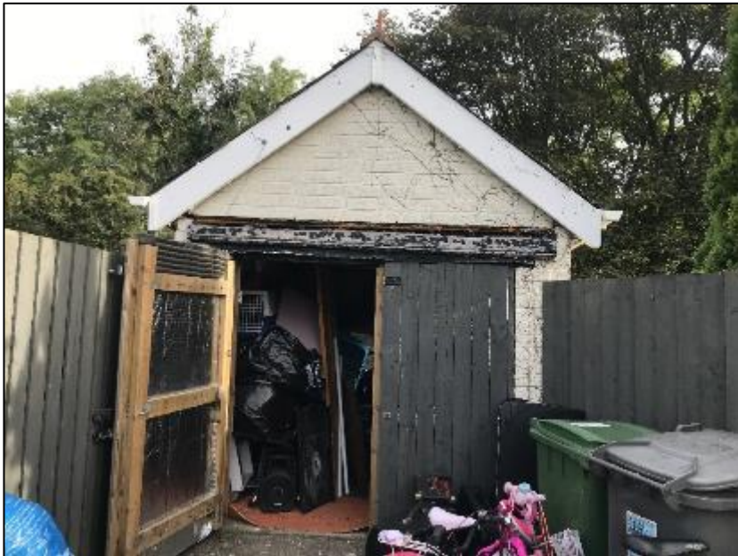
South-western elevation of B2 (pictured above).
