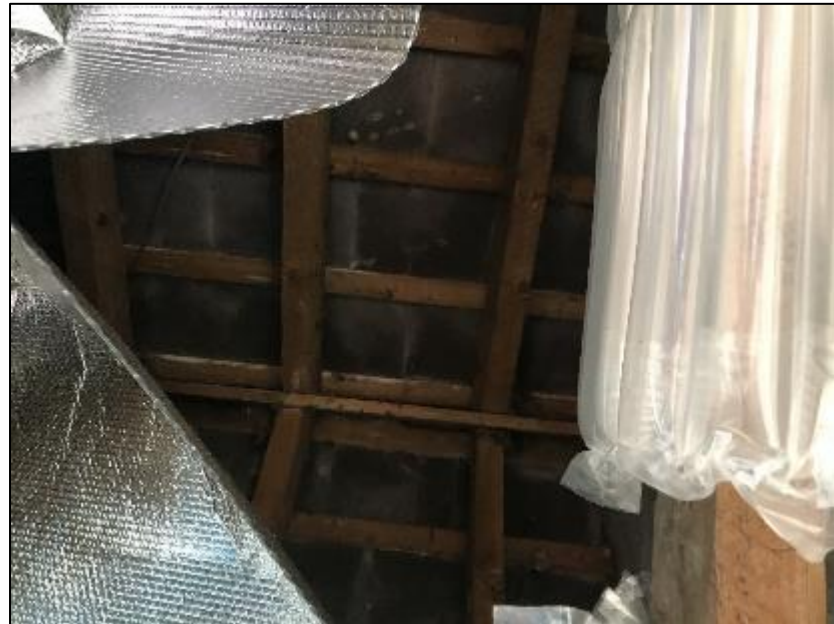
Interior of B2 (pictured above).
