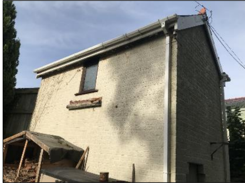
North-eastern and south-eastern elevations of B2 (pictured above).
