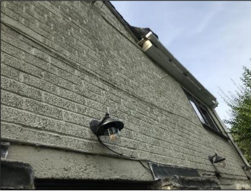
North-eastern elevation of B1 (pictured above).
