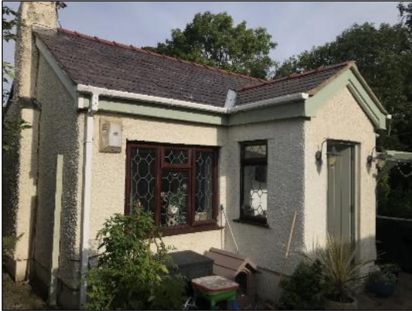
Southern-eastern elevation of B1 (pictured above).
