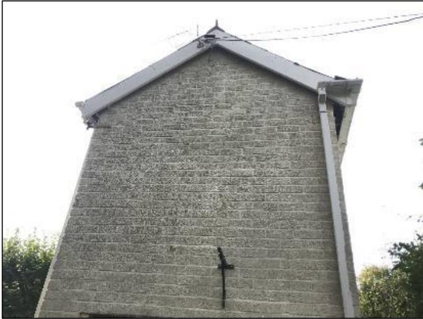
North-eastern gable-end of B2 (pictured above).
