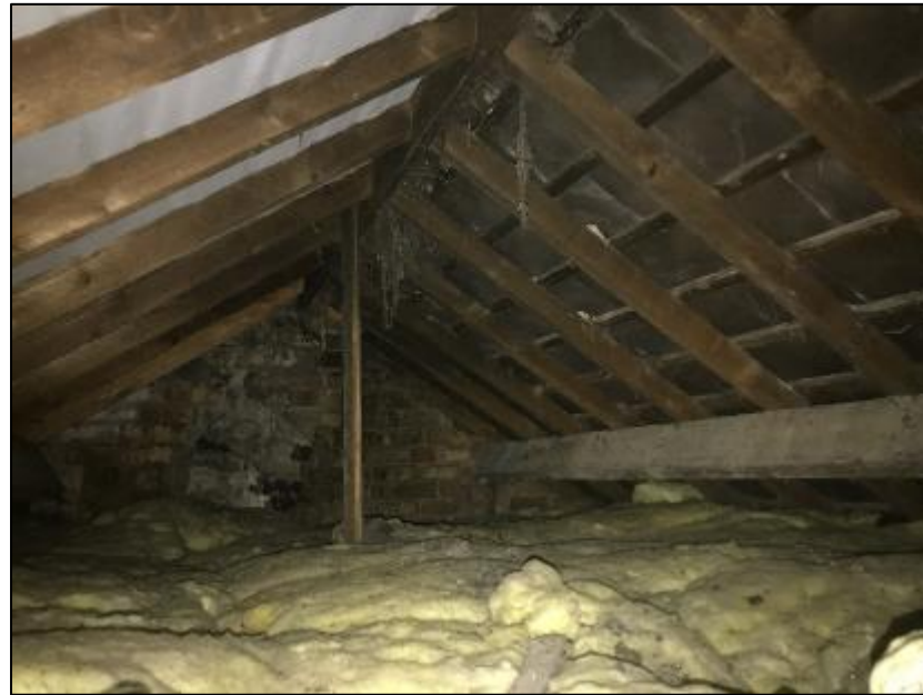
Loft space of B1 (pictured above).
