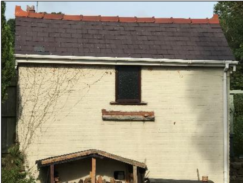
South-eastern elevation of B2 (pictured above).
