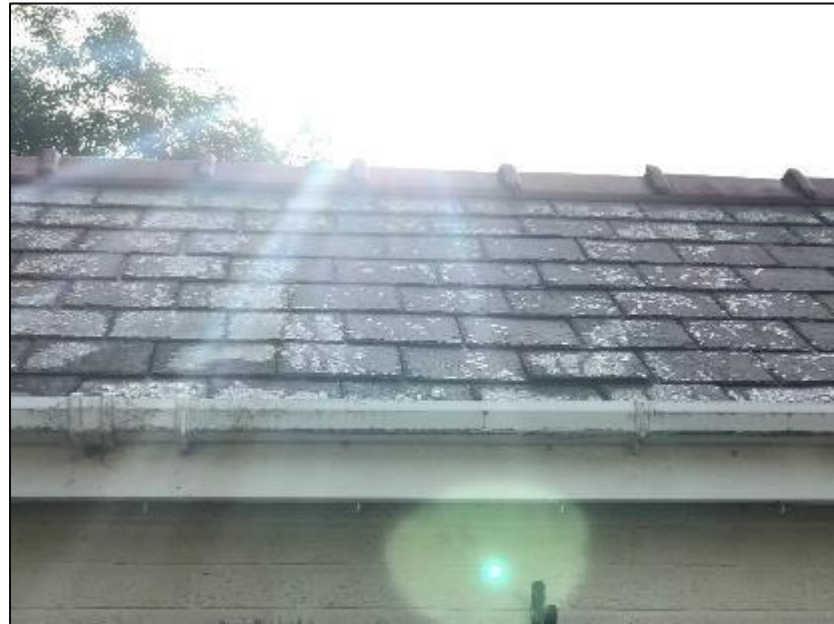
Close-up of roof structure on south-eastern elevation of B2 (pictured above).
