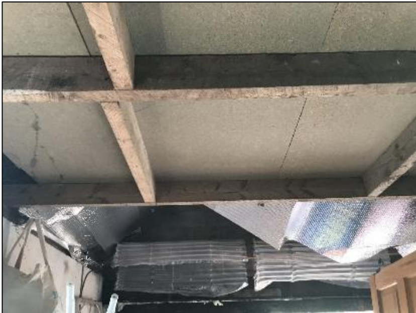
Interior of B2 (pictured above).
