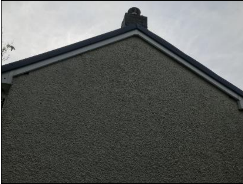
Gable-end on north-western elevation of B1 (pictured above).
