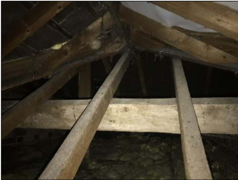
Loft space of B1 (pictured above).
