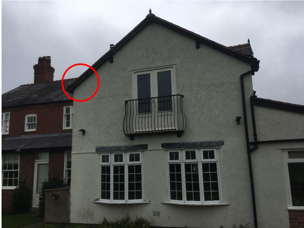
Photograph 2- Fascia Boarding to be removed by hand
