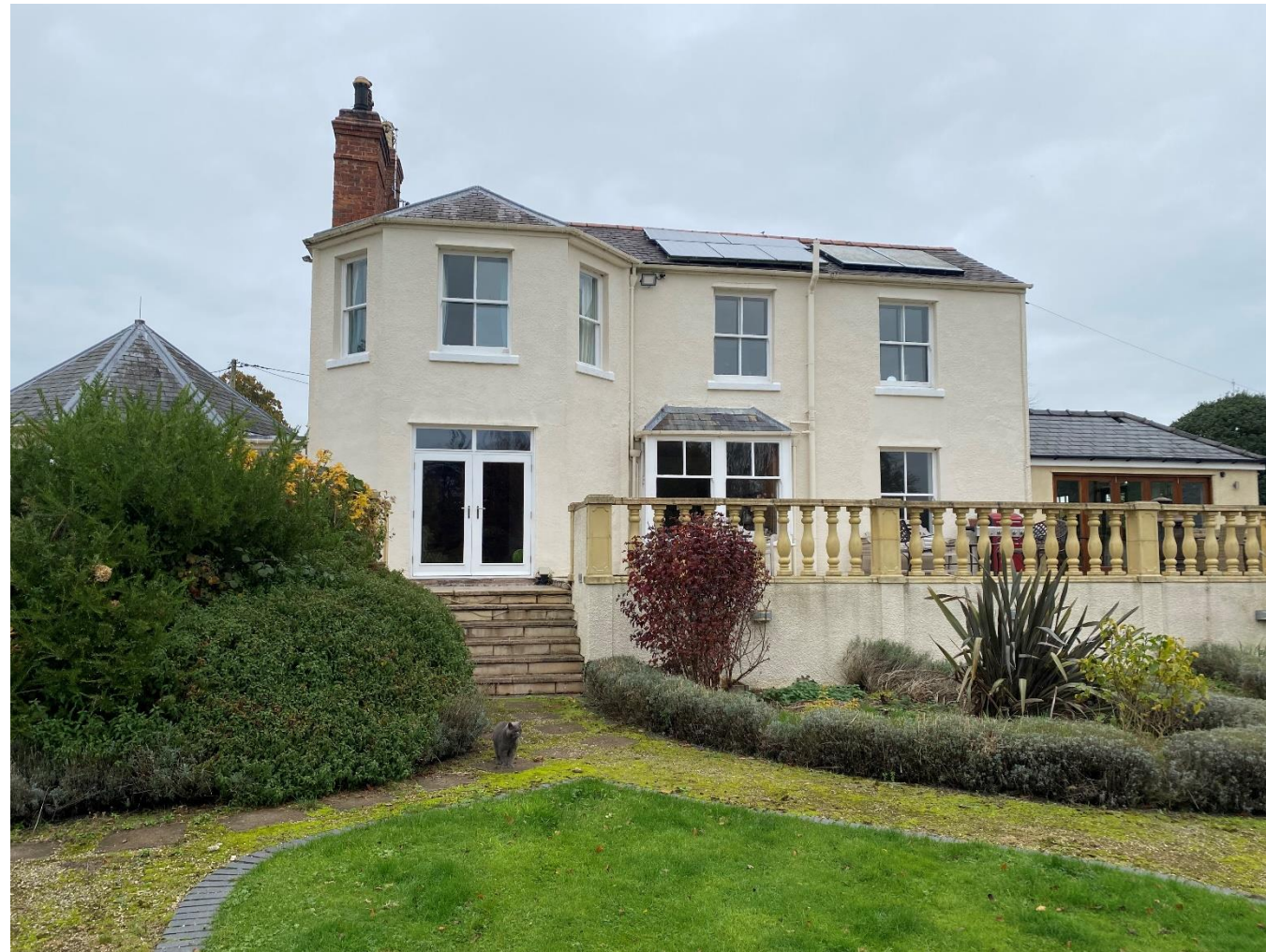
Rear elevation of main Lodge facing rear garden
