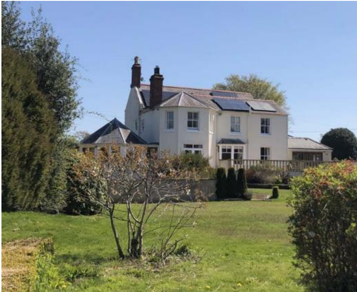
Rear elevation showing conservatory
