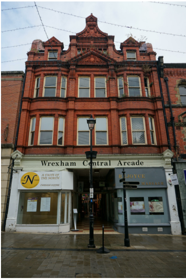
Full elevation of 58 and 58a Hope Street
