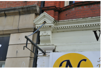
Signage bracket to be replaced
