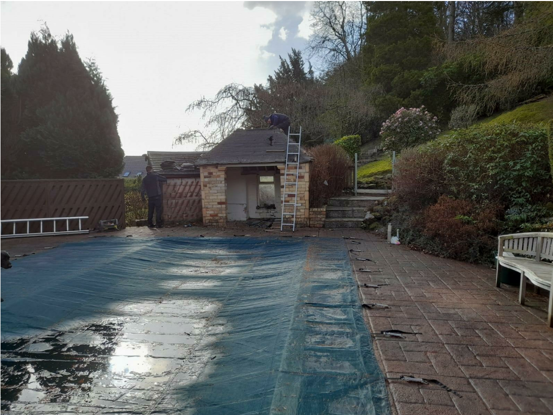
PHOTO 1- Existing Pool House
