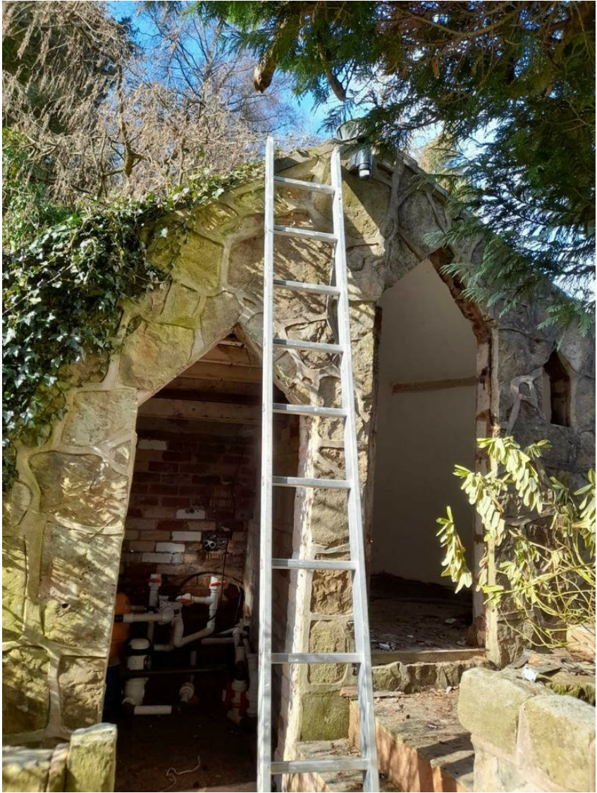
PHOTO 2- Existing Pump House
