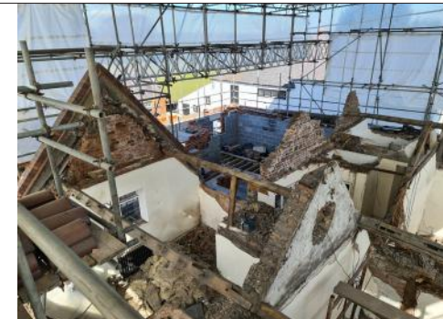
3.12.9 - Bedroom 04- Post Roof Removal
