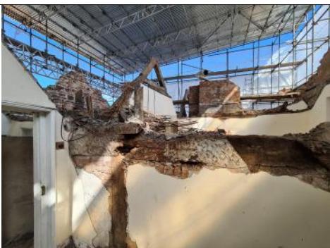
3.9.7 - Master Bedroom- Post Roof Removal
