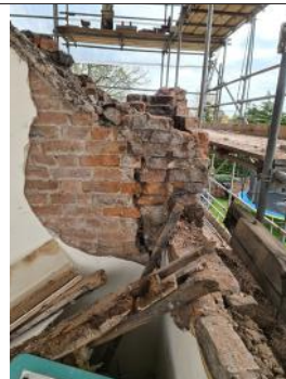
3.12.8 - Bedroom 04- Post Roof Removal
