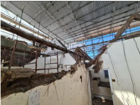
3.10.7 - Bedroom 02- Post Roof Removal
