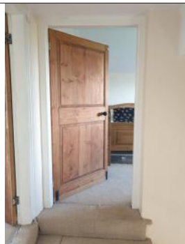
3.13.2 - First Floor Landing
