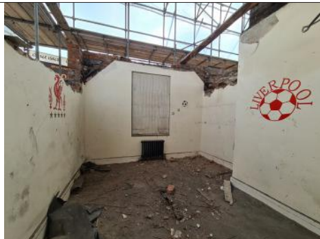
3.11.8 - Bedroom 03- Post Roof Removal
