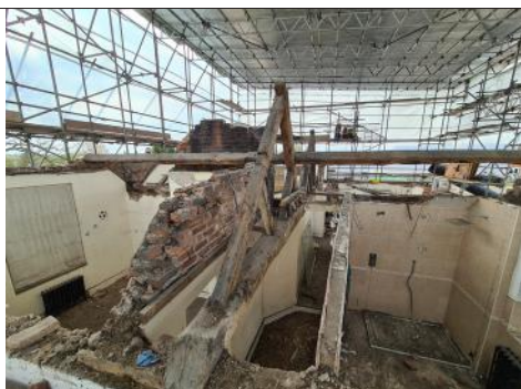
3.14.7- Bathroom- Post Roof Removal
