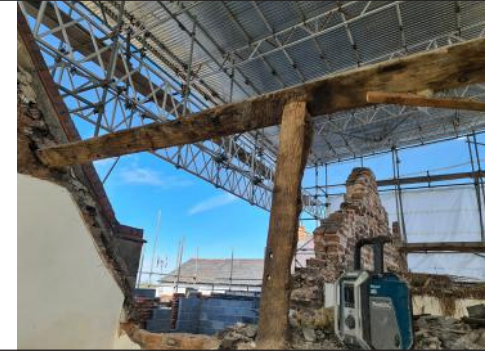
3.12.6 - Bedroom 04- Post Roof Removal
