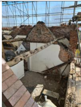
3.12.7 - Bedroom 04- Post Roof Removal
