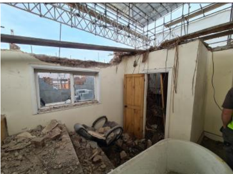
3.13.4 - First Floor Landing- Post Roof Removal
