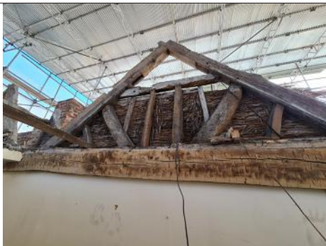
3.13.11 - First Floor Landing- Post Roof Removal
