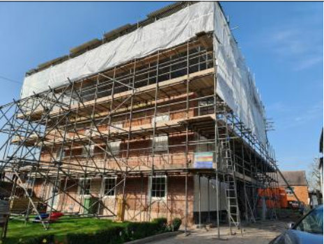
3.1.31 - External- Post Roof Removal
