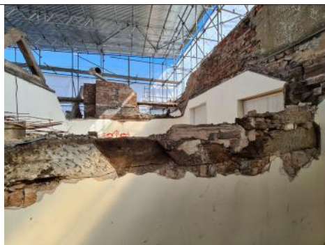
3.9.8 - Master Bedroom- Post Roof Removal
