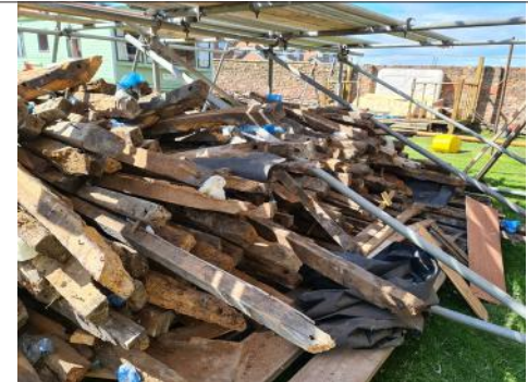
3.1.33 - External- Post Roof Removal
