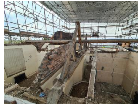
3.13.3 - First Floor Landing- Post Roof Removal
