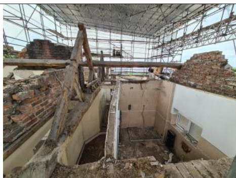
3.14.8 - Bathroom- Post Roof Removal
