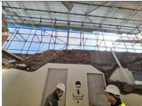
3.10.8 - Bedroom 02- Post Roof Removal
