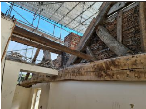
3.13.10 - First Floor Landing- Post Roof Removal
