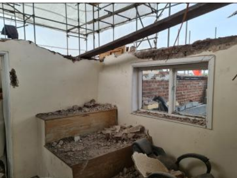
3.13.5 - First Floor Landing- Post Roof Removal
