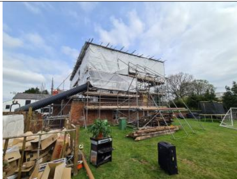
3.1.32 - External- Post Roof Removal
