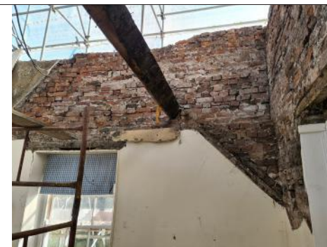
3.9.9 - Master Bedroom- Post Roof Removal
