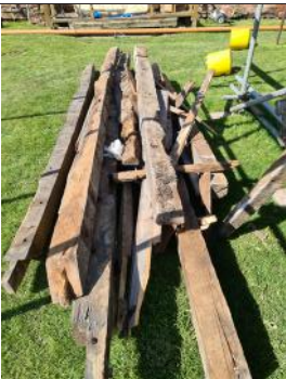
3.1.34 - External- Post Roof Removal
