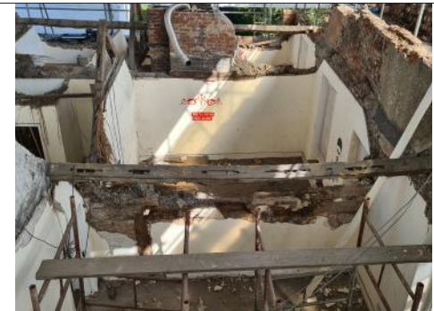
3.10.9 - Bedroom 02- Post Roof Removal
