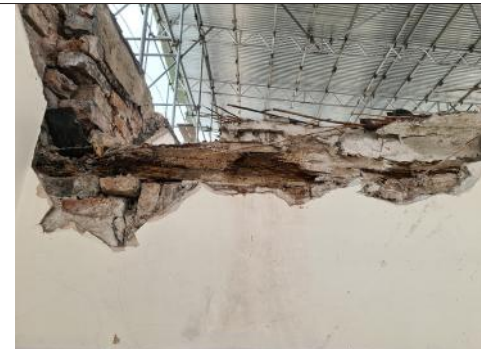
3.11.9 - Bedroom 03- Post Roof Removal
