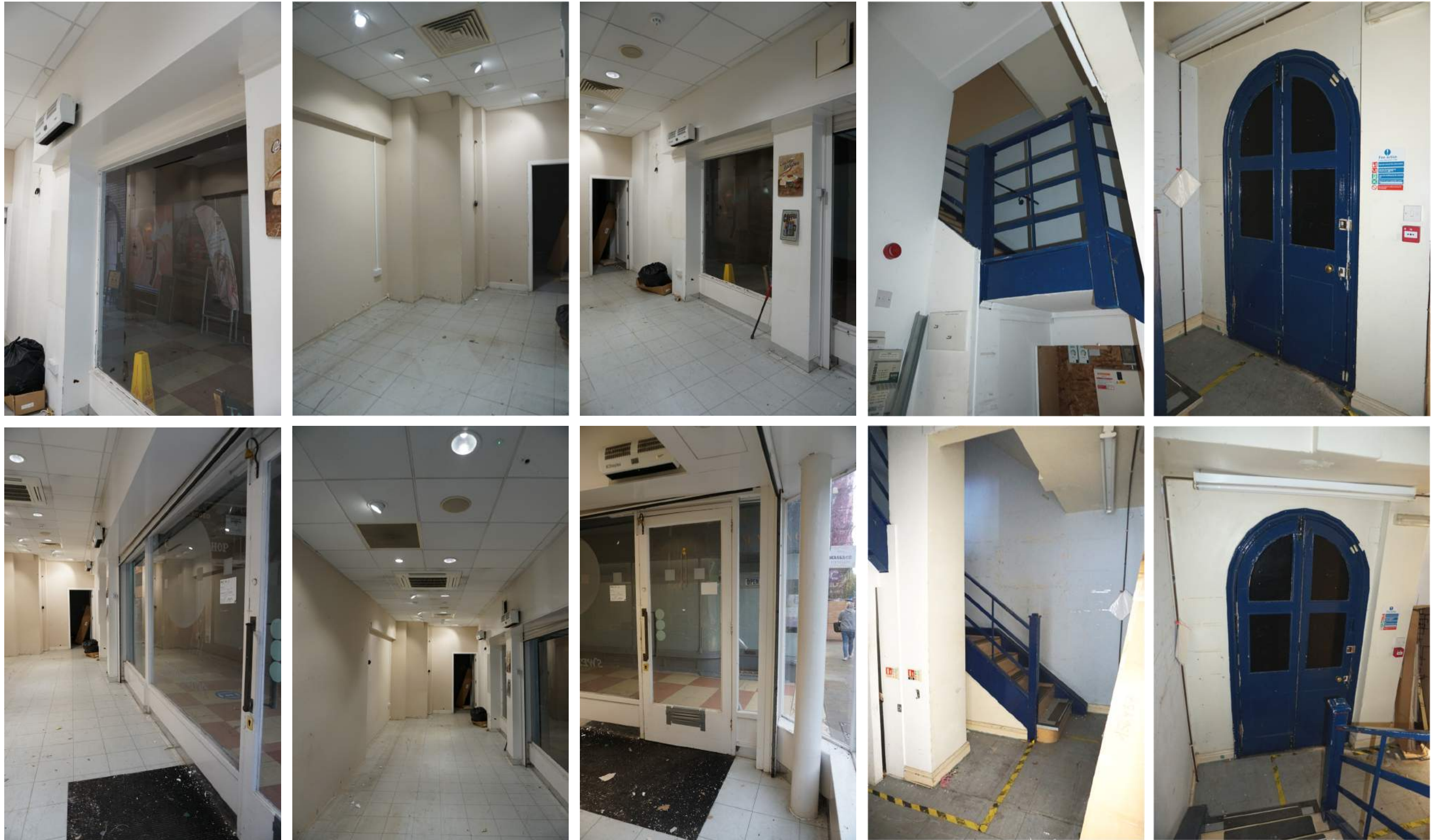
EXISTING GROUND FLOOR PHOTOGRAPHS
