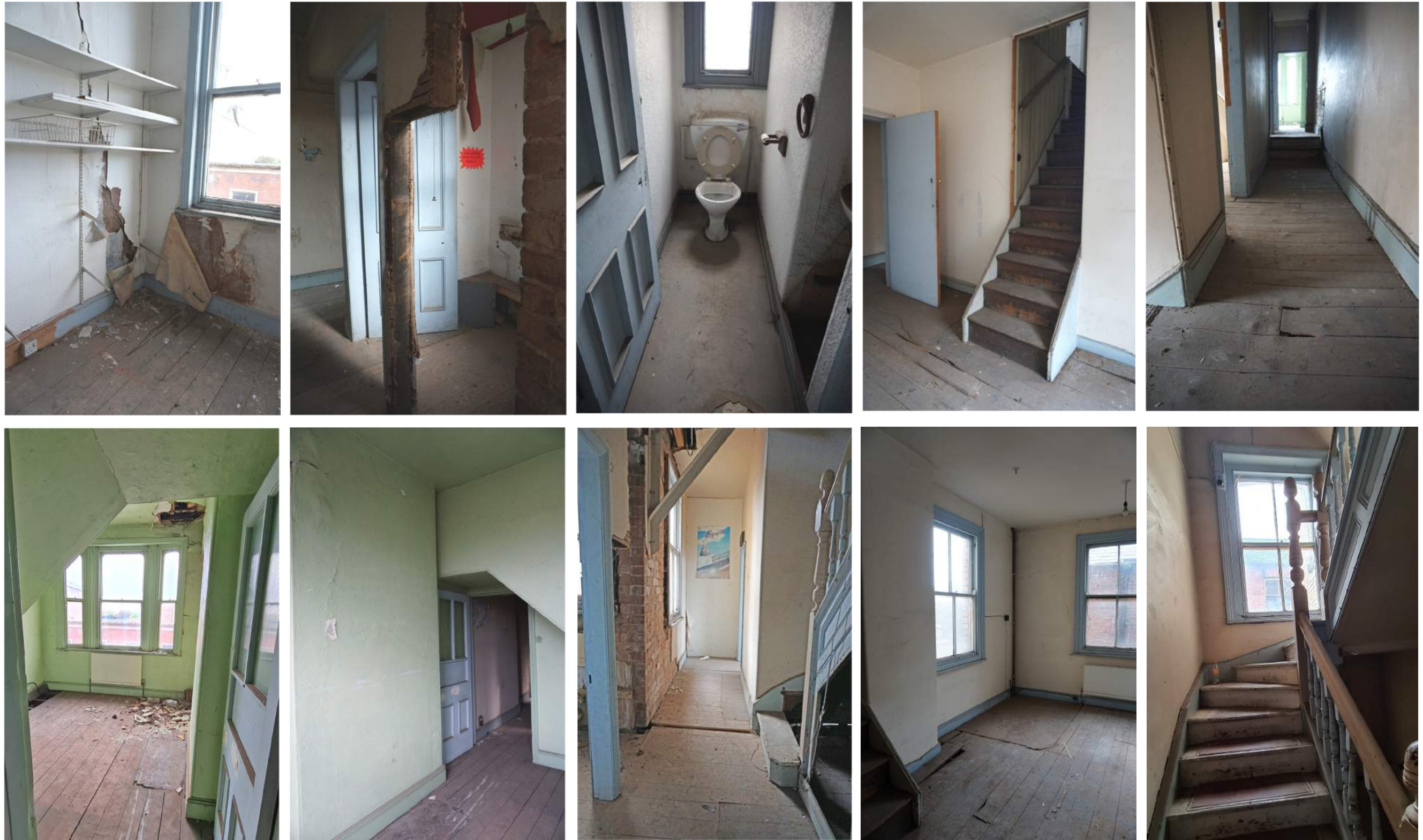
EXISTING SECOND FLOOR PHOTOGRAPHS
