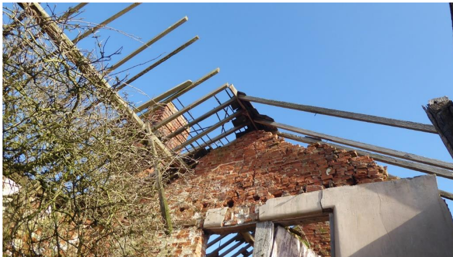
Figure 4.4. Internal view of building 1
