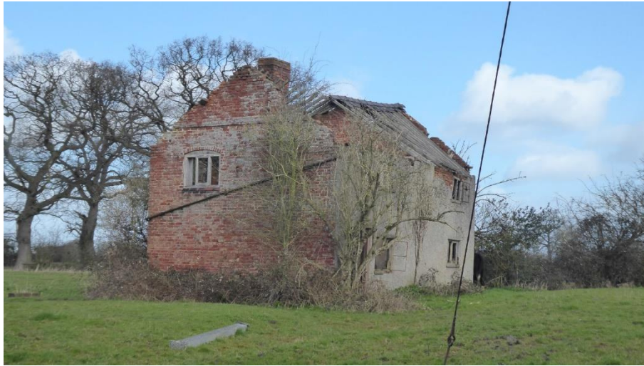
Figure 4.3. Building 1 from south
