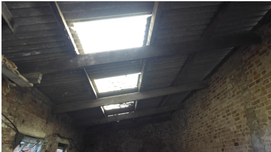
Figure 4.8. Internal view of building 3
