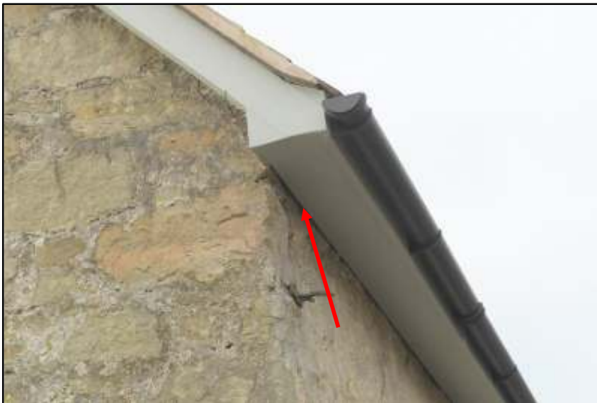
Gaps along the soffits at the rear
