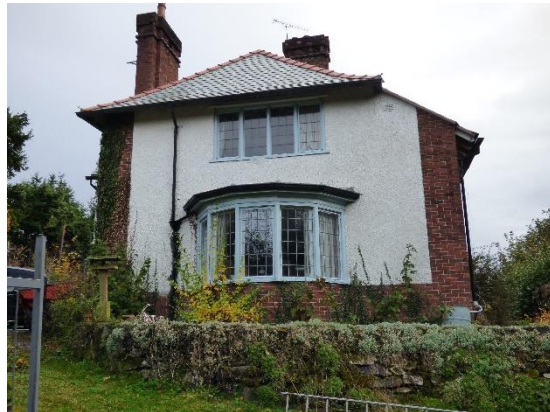
West elevation and walkway
