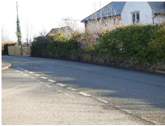
New gate and temporary fence 1/2/22
