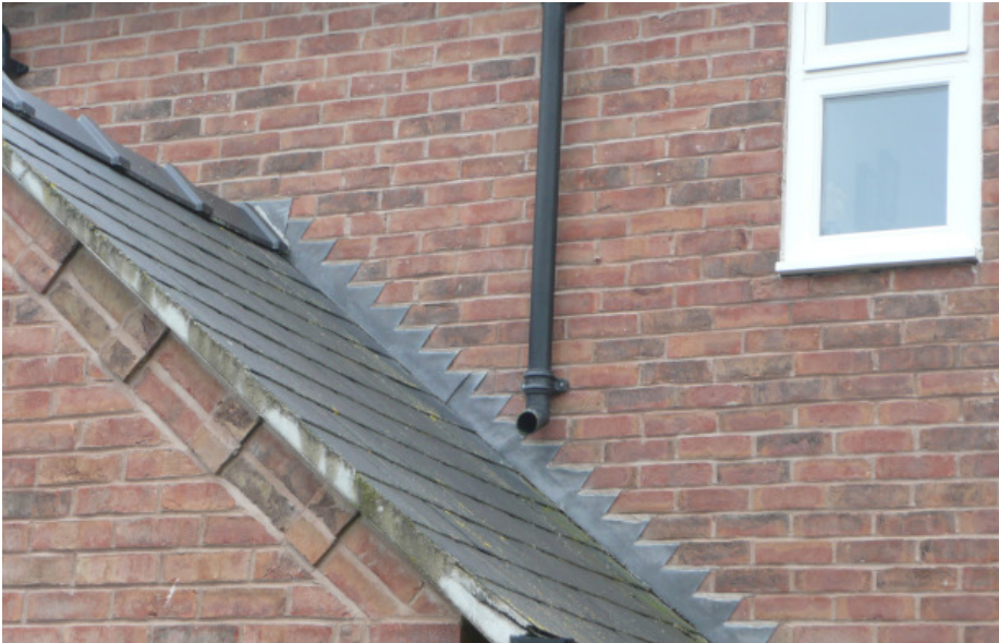
Gable verge brickwork detail
