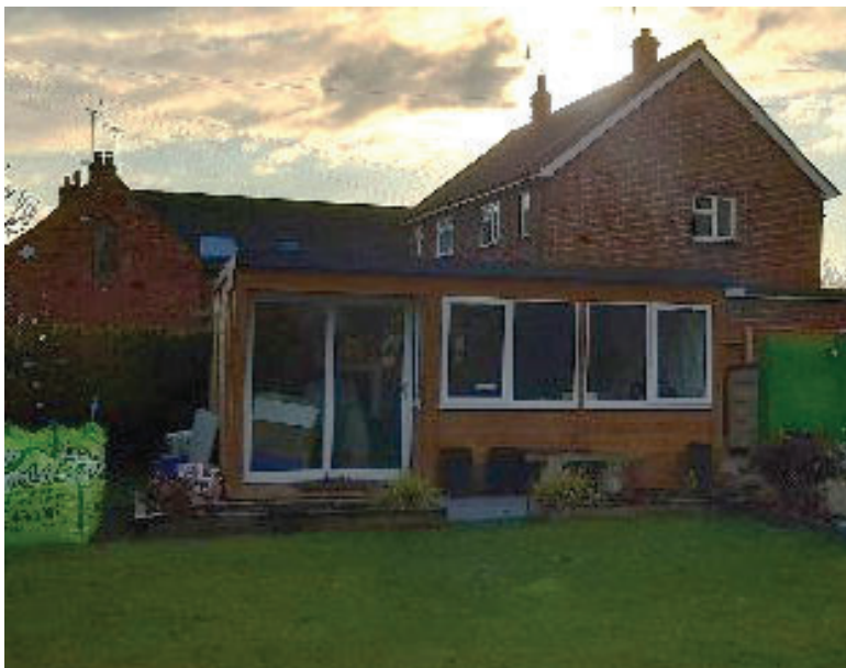
Figure 4 – Outbuilding and wall viewed from within the garden.
