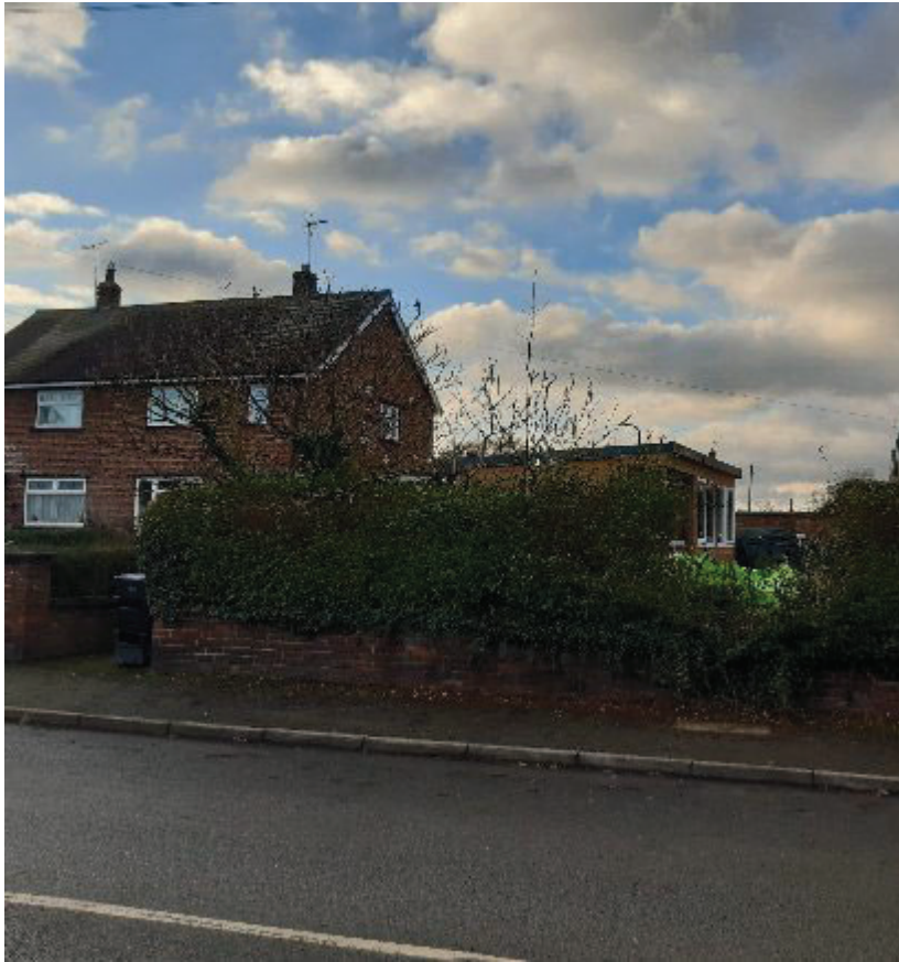
Figure 3 – Outbuilding viewed from Bridge Street.
