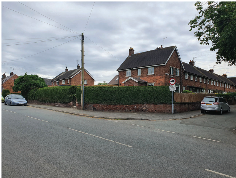
Figure 2- Site when viewed from Bridge Street.
