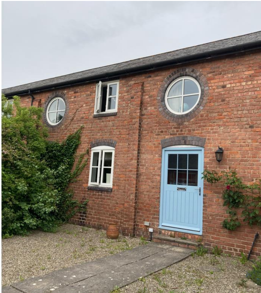
Fig. 2 – Picture of Existing Front Elevation
