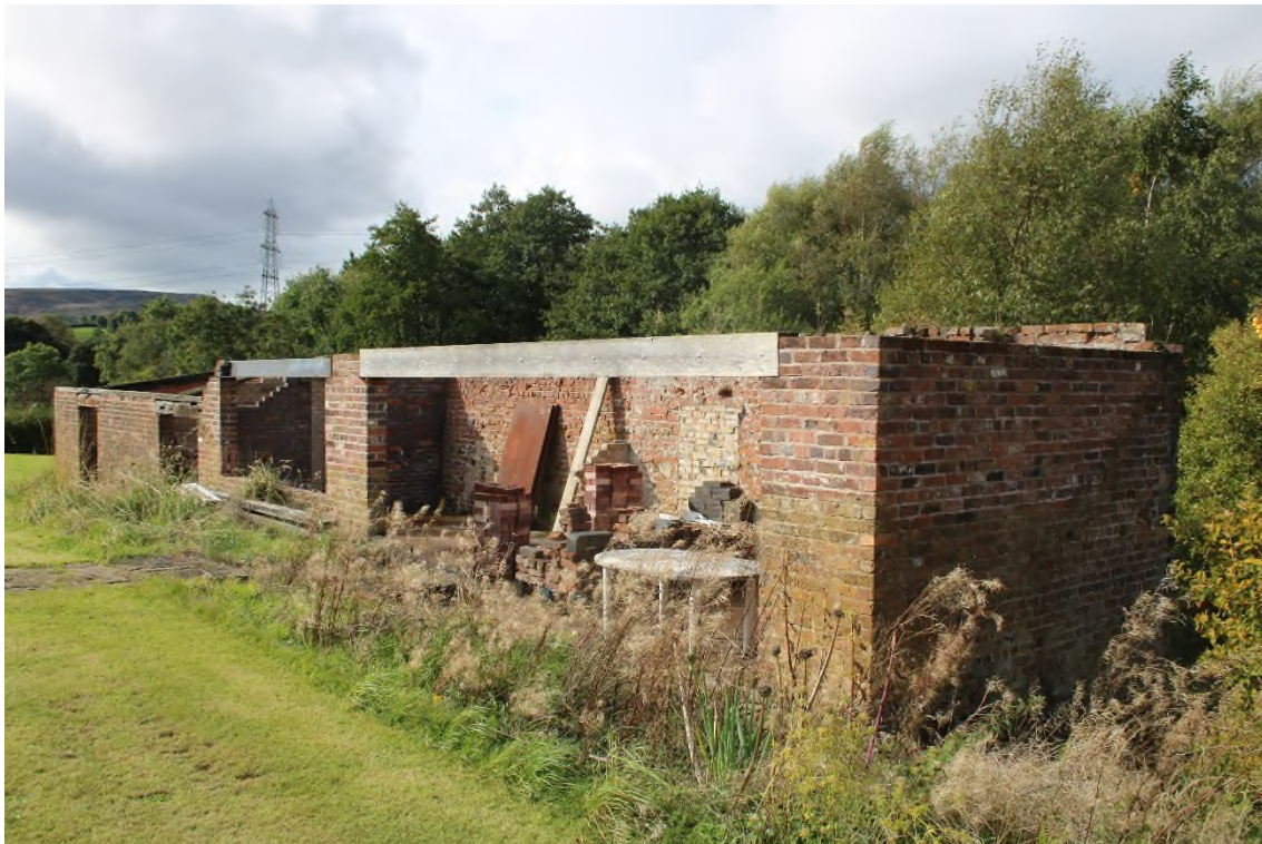
Photo 1 – Outbuilding Looking North West
