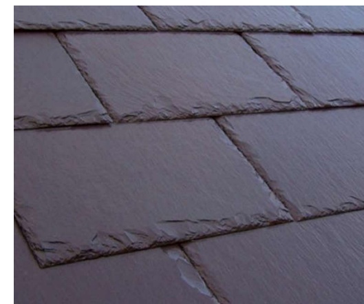
Natural Welsh Slate Roof
