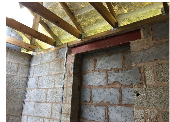
Remedial works to structural openings
