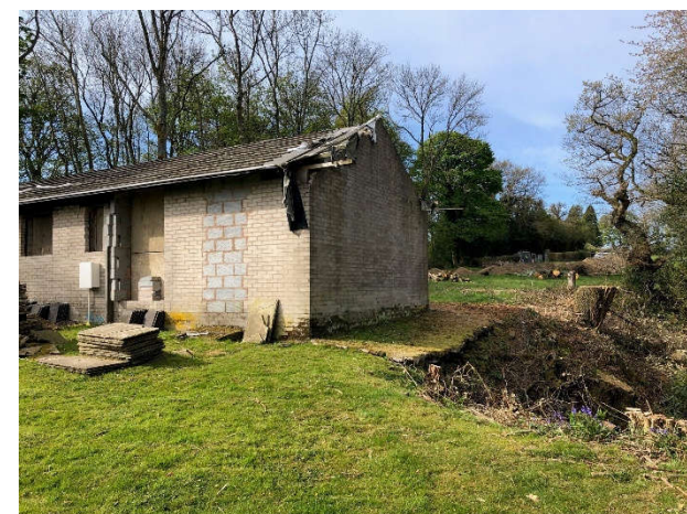
Elevated northwest gable end
