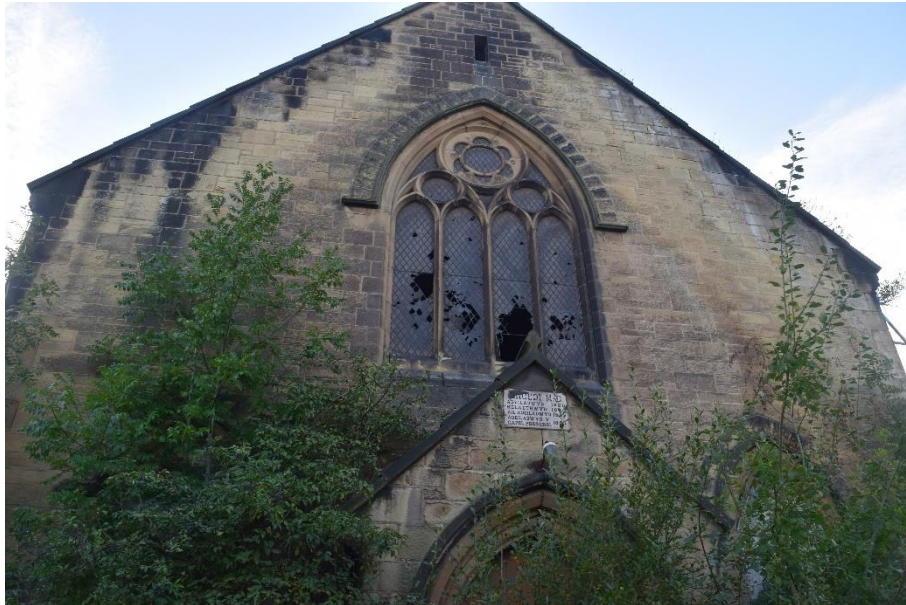
Figure 4.3. Openings in eastern window
