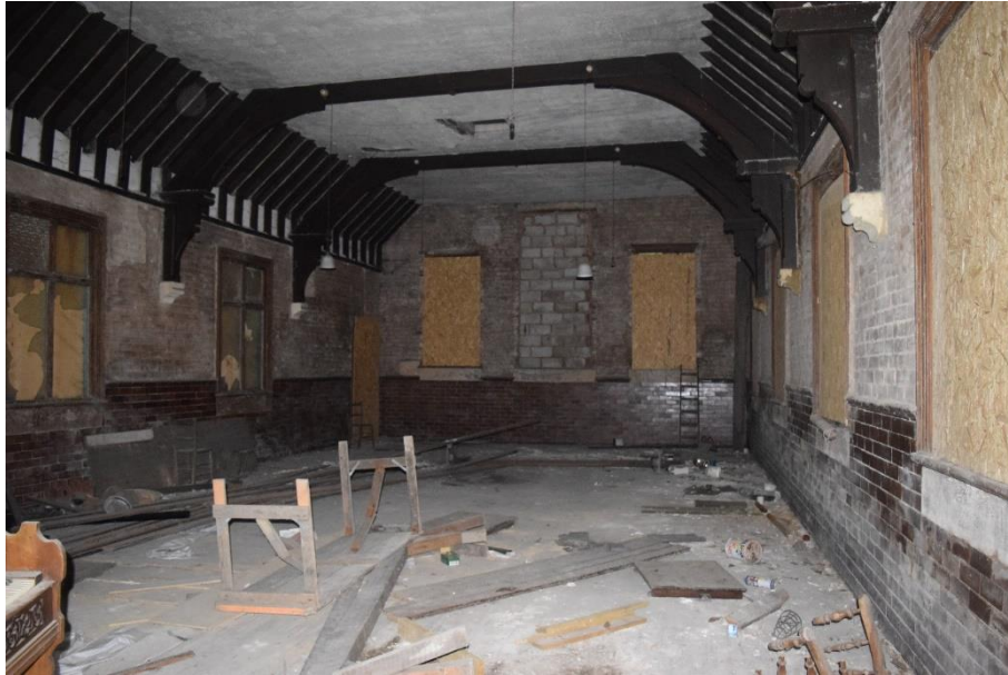
Figure 4.5. Interior of school room
