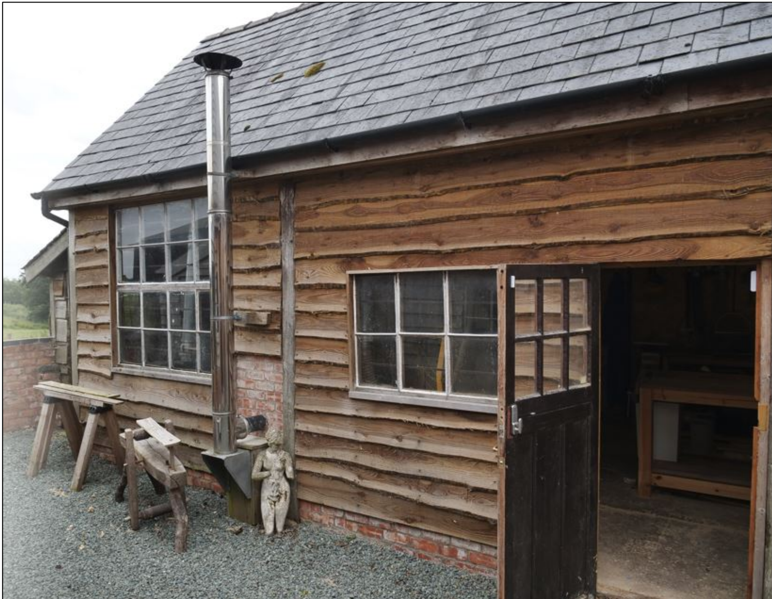
Figure 19: View of Outbuilding 2 Northern Elevation
