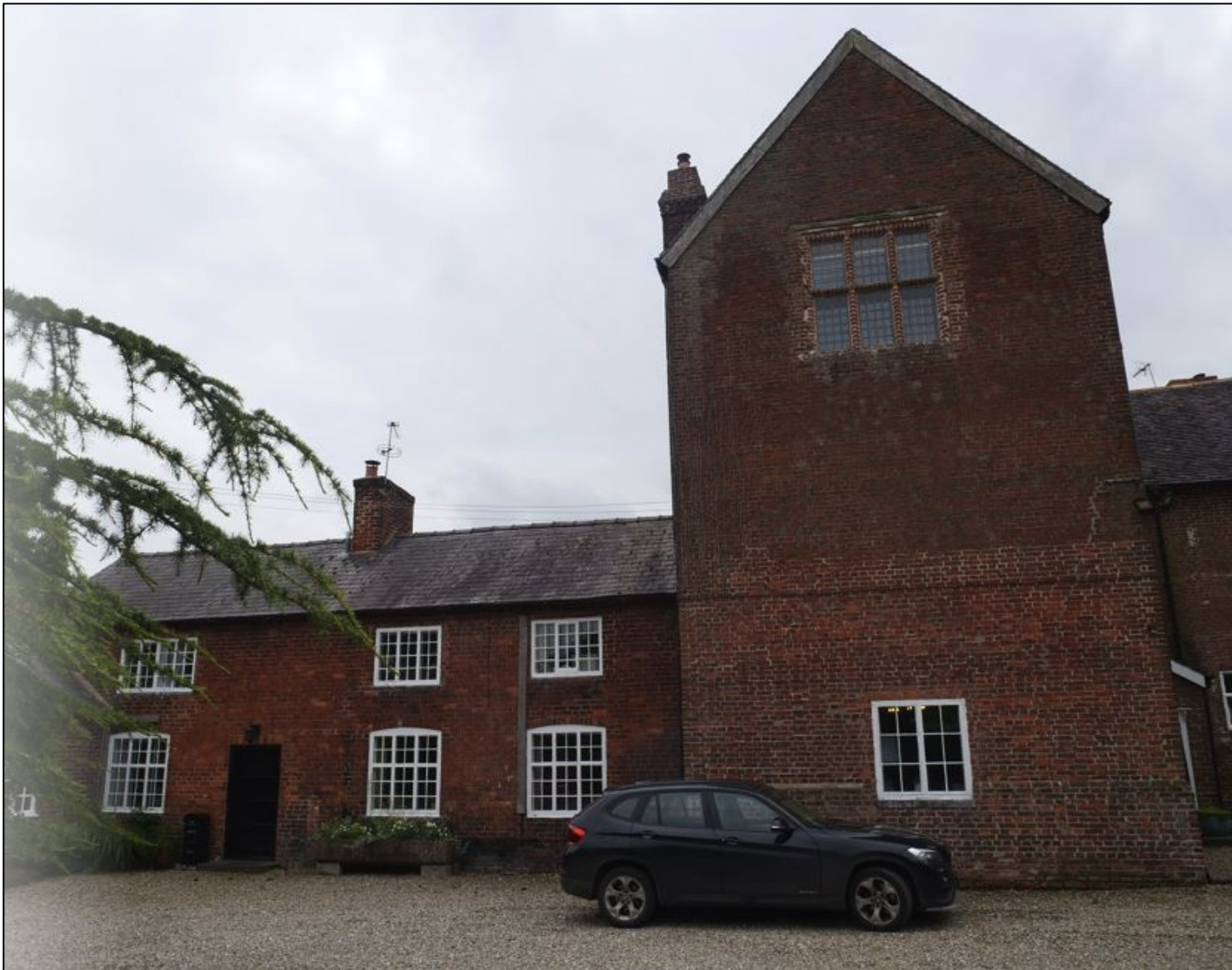
Figure 8: View of North Elevation of Main Hall
