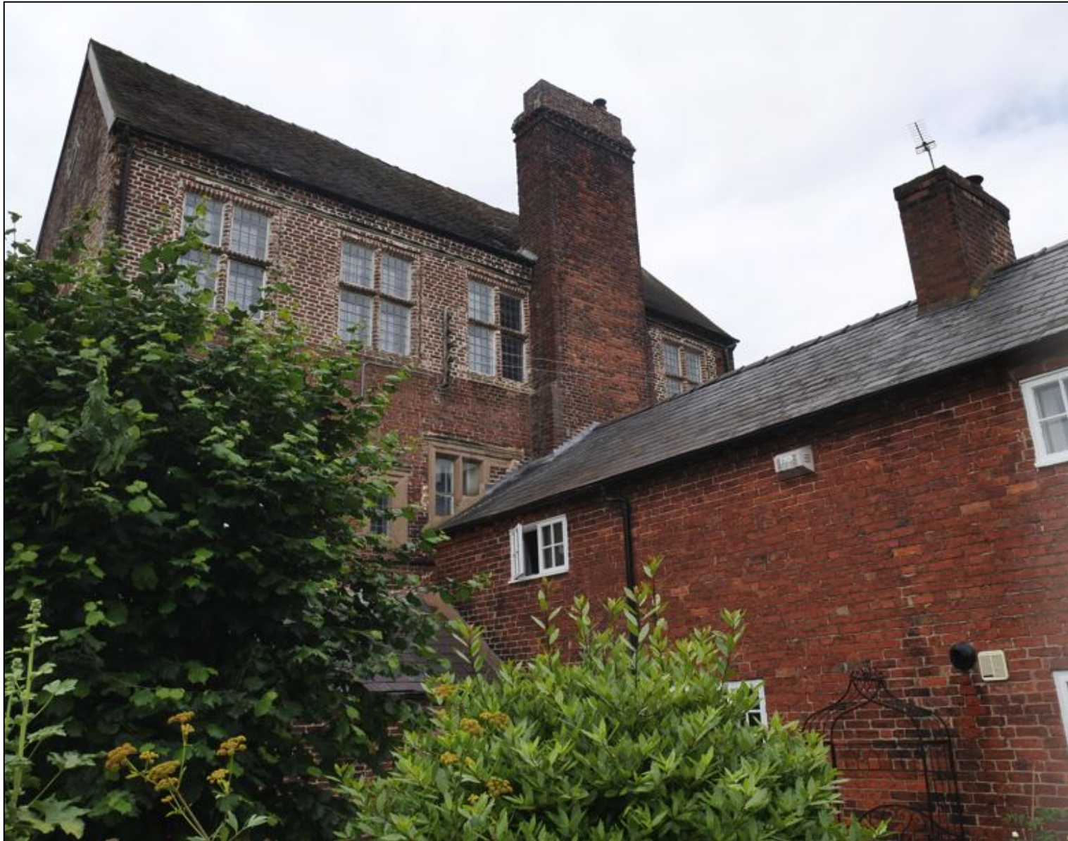
Figure 12: View of East Side Elevation
