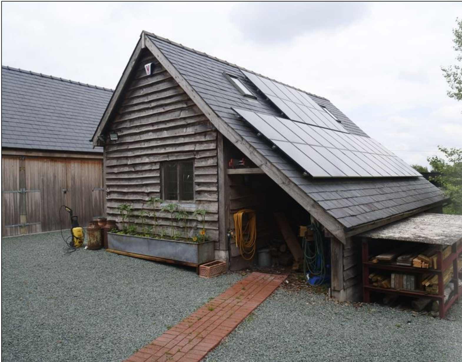
Figure 18: View of Outbuilding 2 Western Gable
