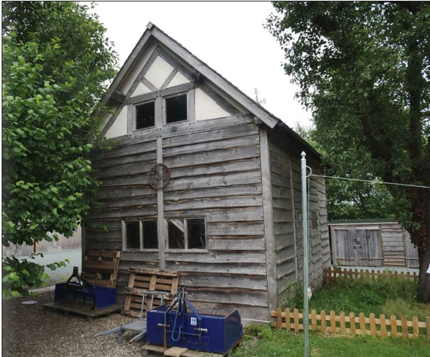
Figure 15: Outbuilding 3 Western Gable
