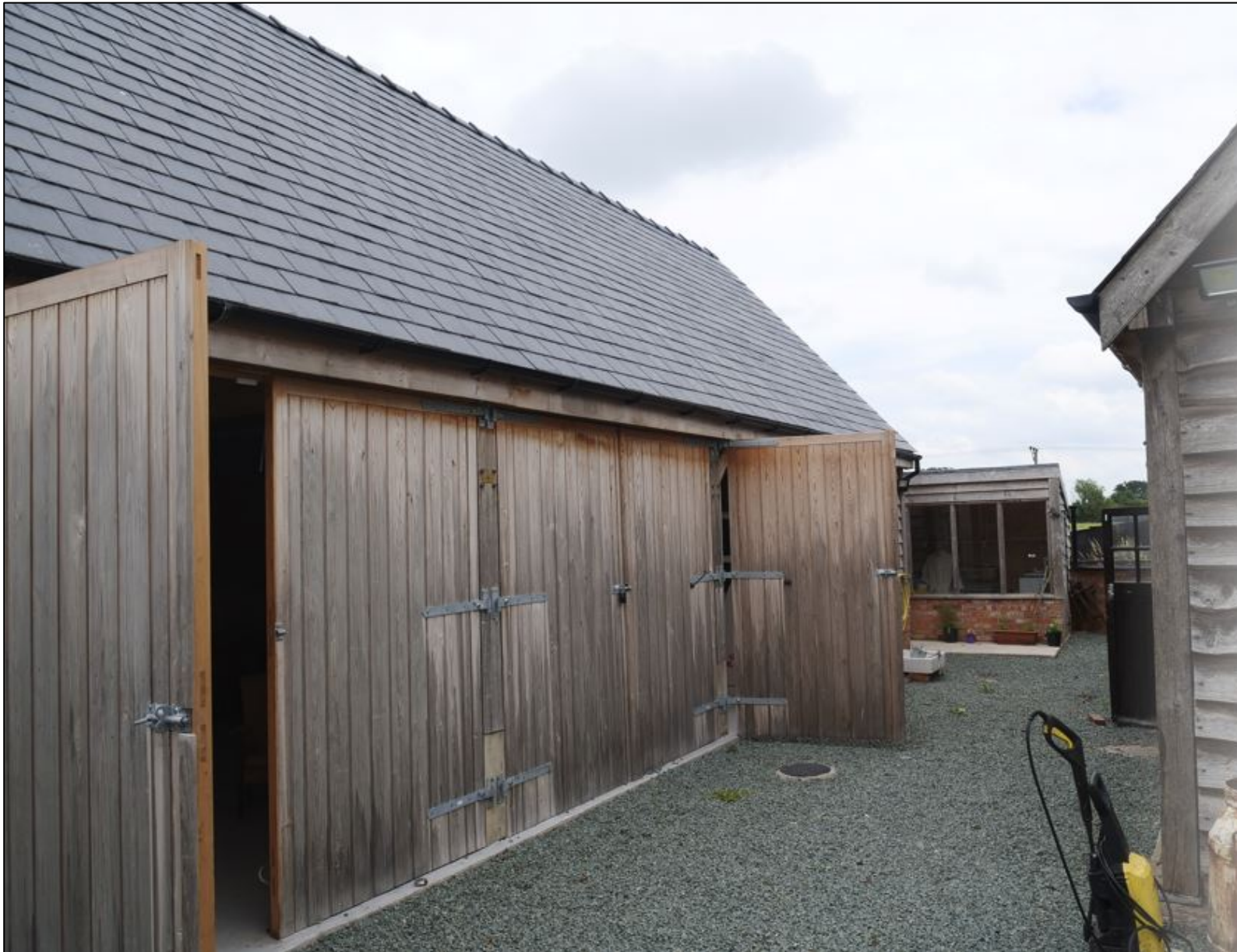
Figure 21: View of Outbuilding 1 Southern Elevation
