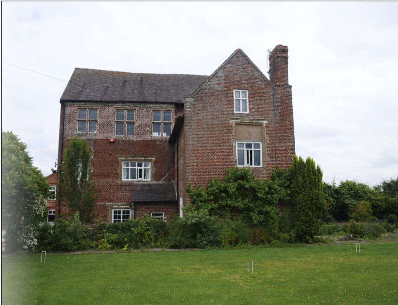
Figure 7: View of South Elevation of Main Hall
