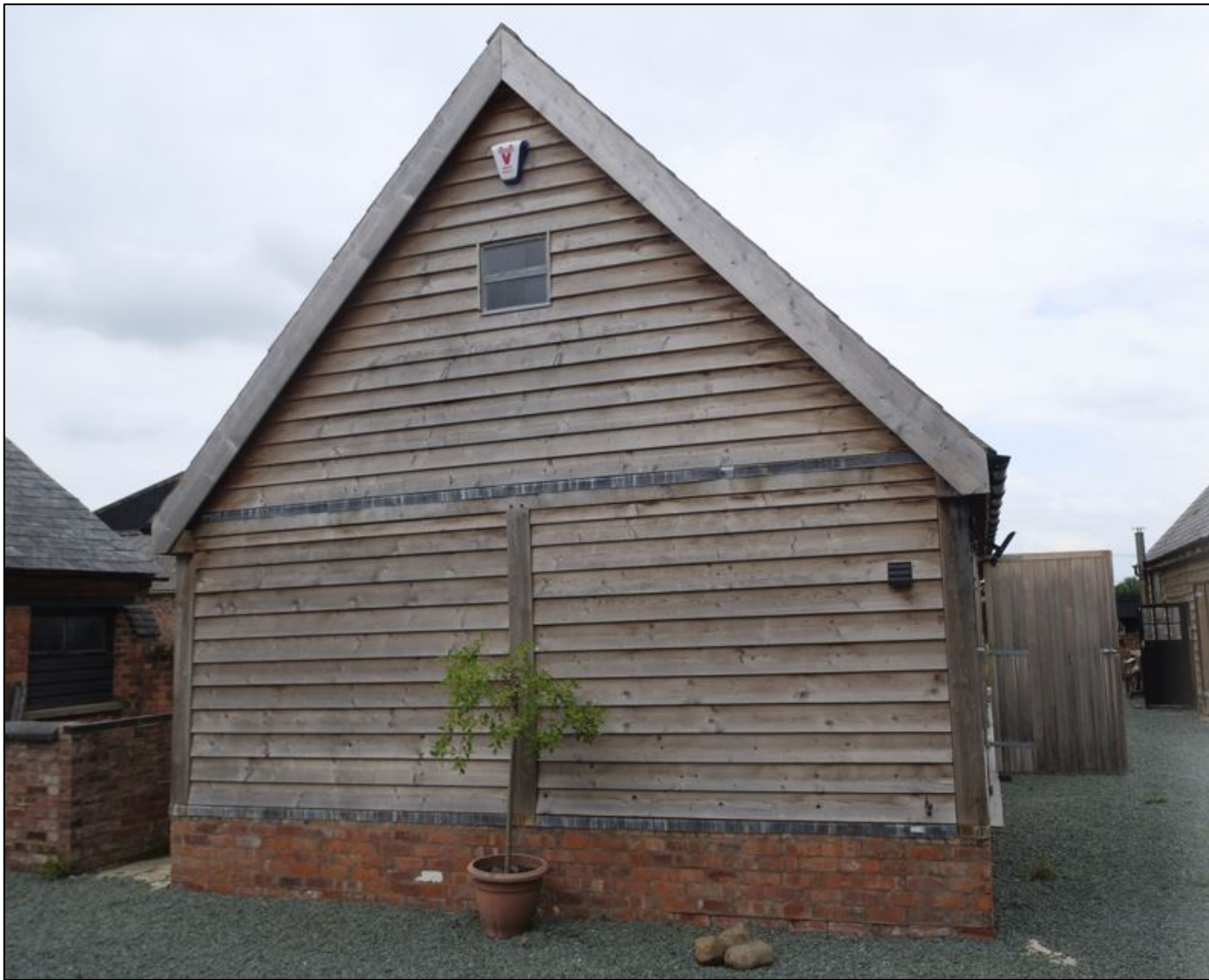
Figure 24: View of Western Gable of Outbuilding 1
