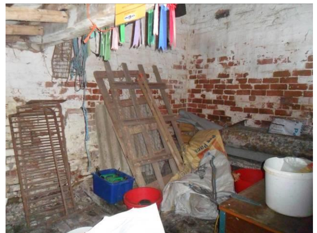
Interior - lean to at the south western elevation
