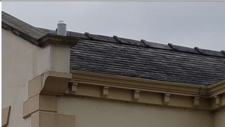
Detail of roof, verge and eave design
