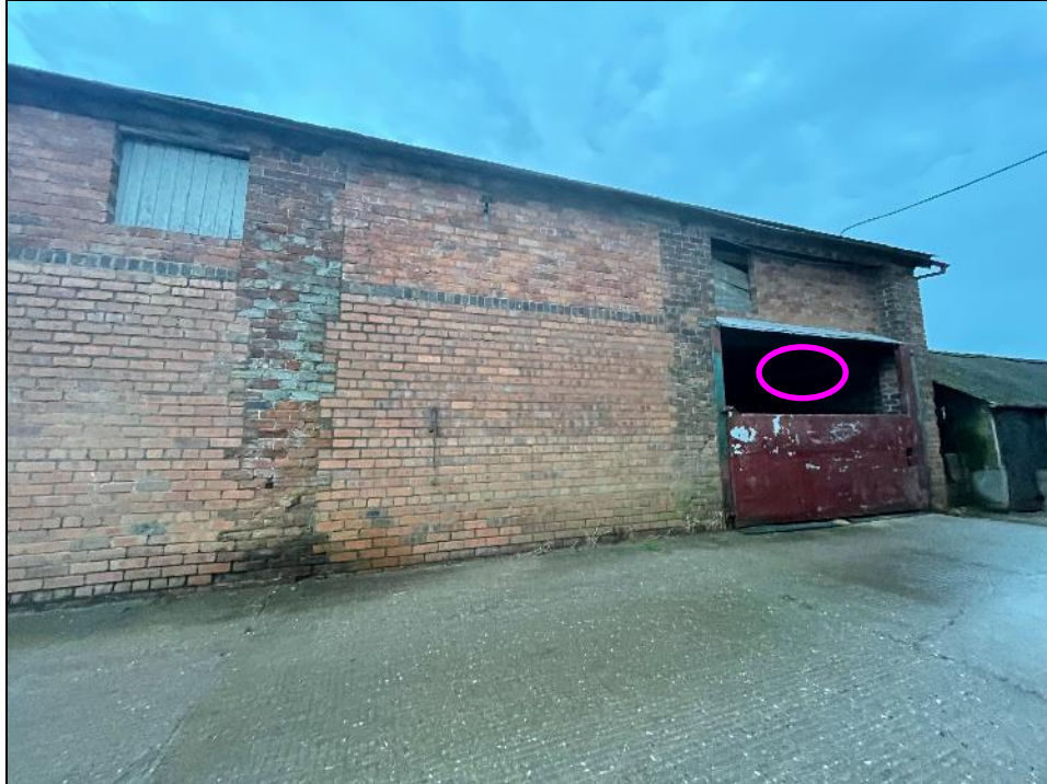
Plate 3 - Emergence area - Emergence of one Soprano Pipistrelle bat from a ground floor opening 'stable' in the north-western aspect of the barn. During dusk survey 2.
