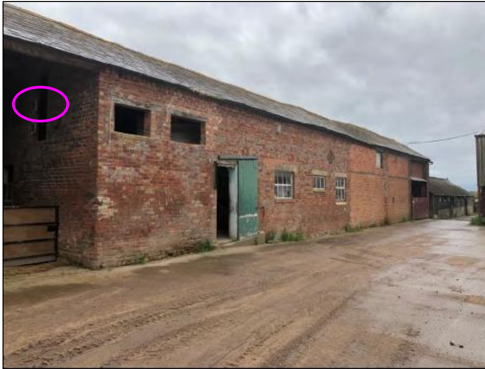
Plate 1 - Emergence area - The central purpose-built open area facing north-west with access openings to the mezzanine. During dusk surveys 1 and 2.
