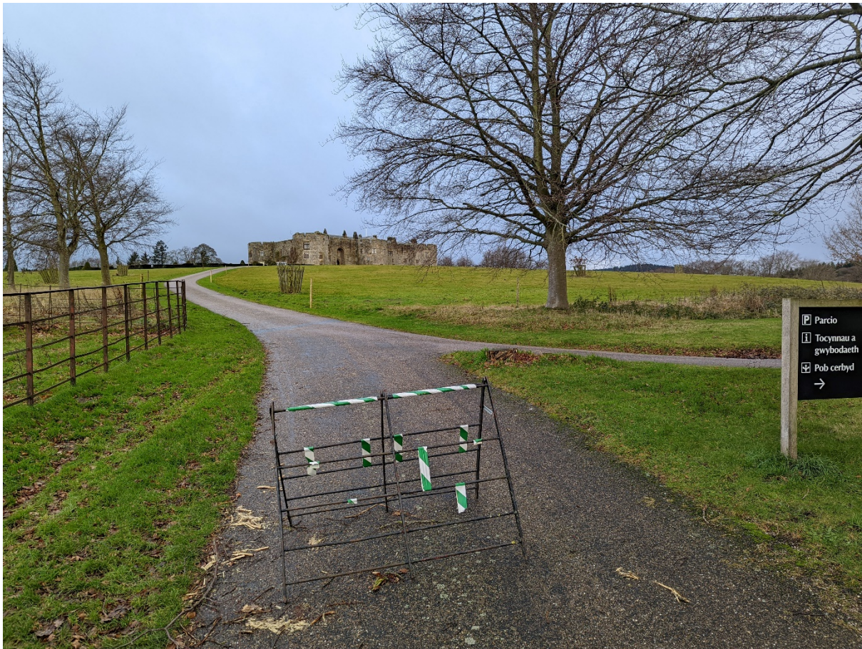
Figure 1: Chirk Castle approach road with current temporary barrier in place at position proposed for removable bollards.
