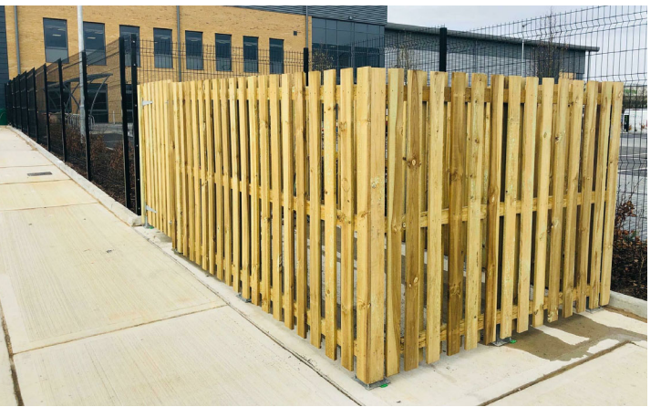
Image: Timber close boarded fence
