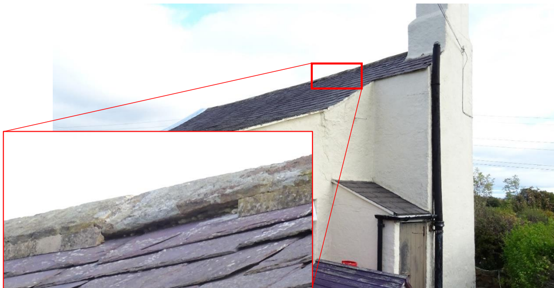
Figure 4.5. Example gap under ridge
