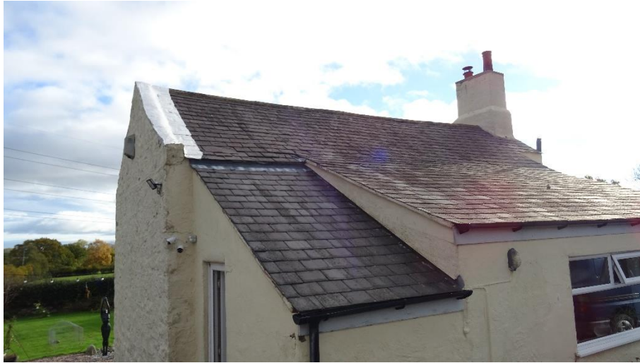
Figure 4.2. Slate tile roof at the west of the property
