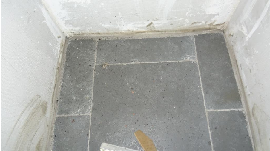
Figure 4.7. Floor beneath chimney
