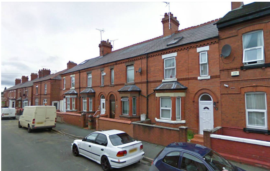
3. Houses on Maesgwyn Road
