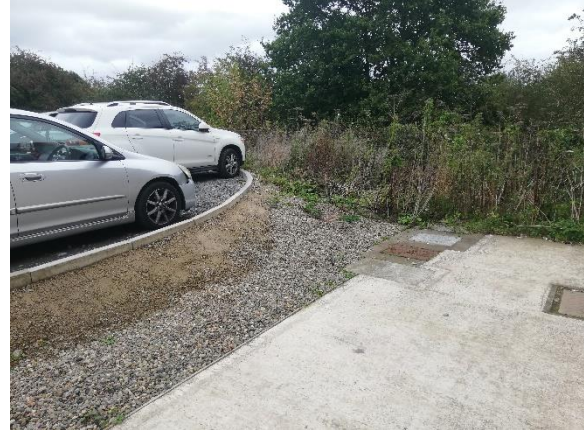
Figure 6. South-eastern Location (camera NE facing) (3)
