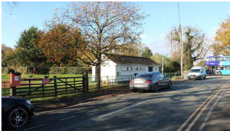
A view to the existing building from The Green
