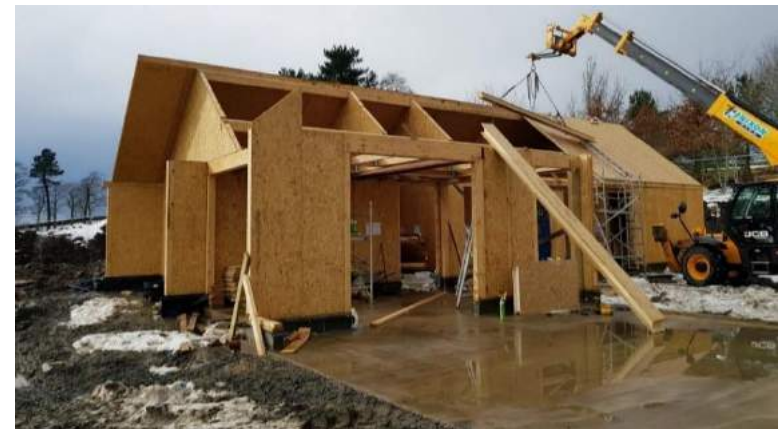
SIPS Construction On-Site (Courtesy of Great Space Architects)
