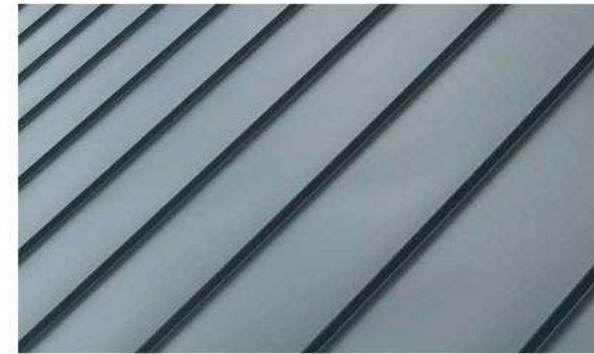
STEEL STANDING SEAM ROOFING
