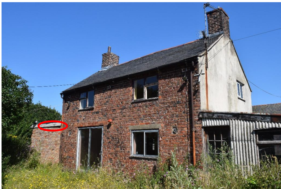
Figure 4.5. Southern elevation of cottage
