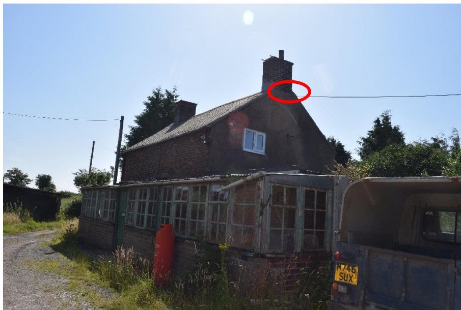
Figure 4.7. Showing emergence point
