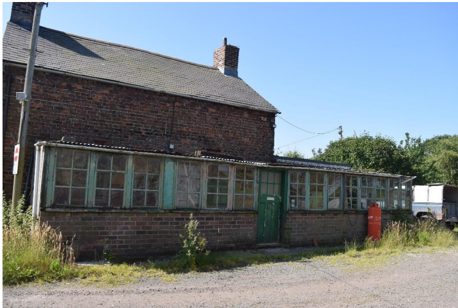
Figure 4.2. Northern elevation of cottage
