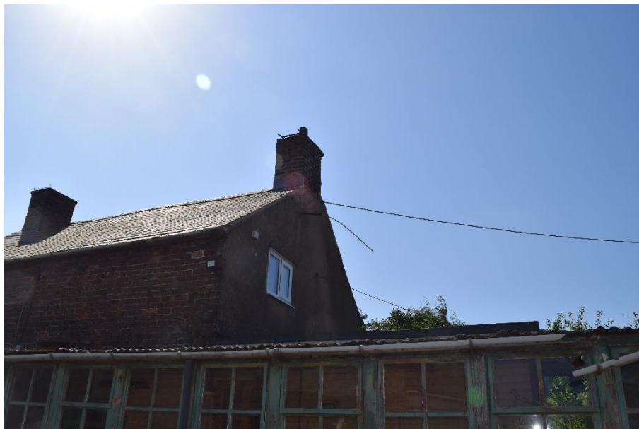
Figure 4.3. western elevation of cottage
