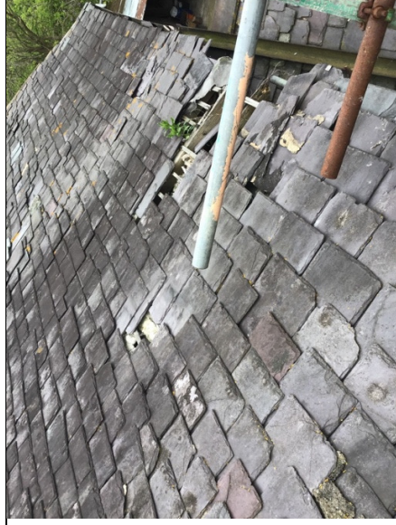
Plate 5: Roof – back of house
