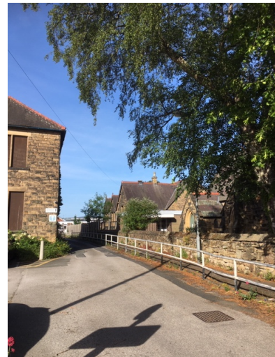
T3 and T4 overhang to site
