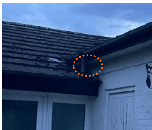
Figure 5.5 - Visual Aid - Emergence location at the roof verge/wall-plate where the eastern wing meets the southern wing of the bungalow from which two Common Pipistrelle emerged during dusk survey 2
