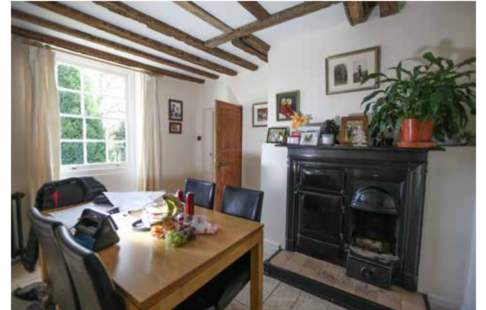
Plate 45 above: Ground floor Dining Room, with 20th century kitchen range inserted into 18th century chimney breast.
