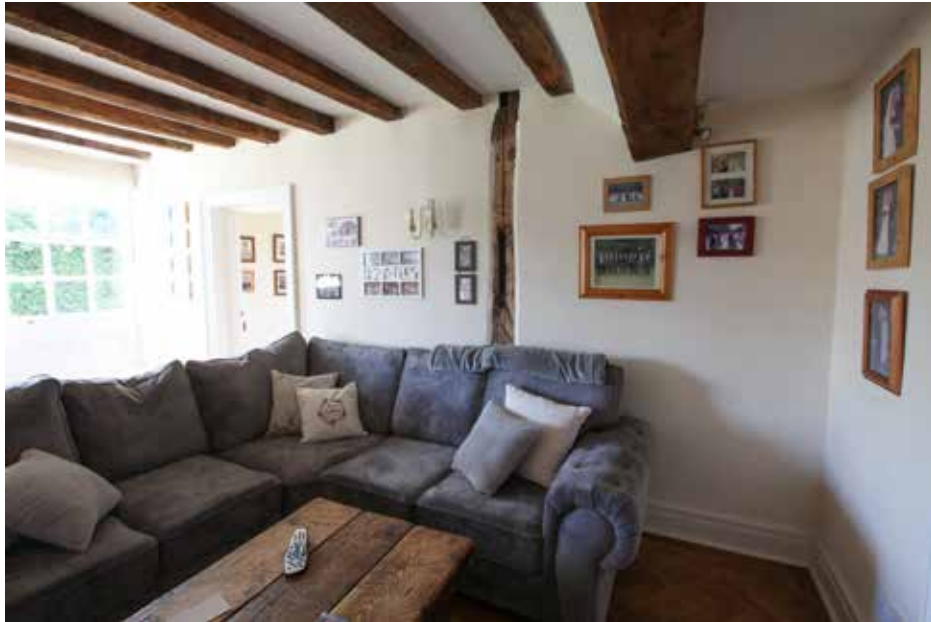
Plate 48 above: Former hall, with post in-situ.
