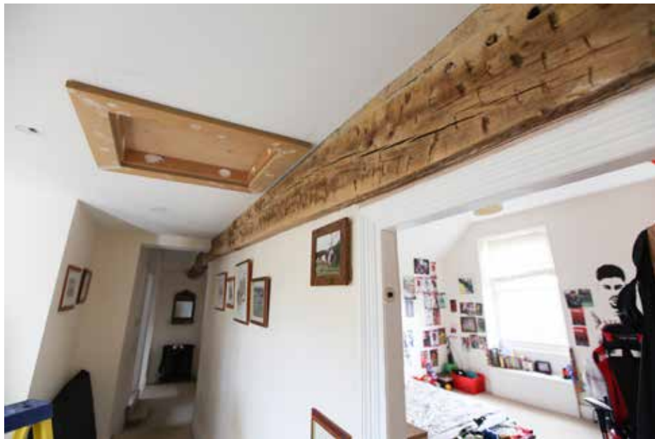
Plate 34 above: Long beam of ca. 1700 supporting pair of Queen strut trusses. Plate 35 below: Bedroom 2 with raised soffit to ceiling of ca. 1730.
