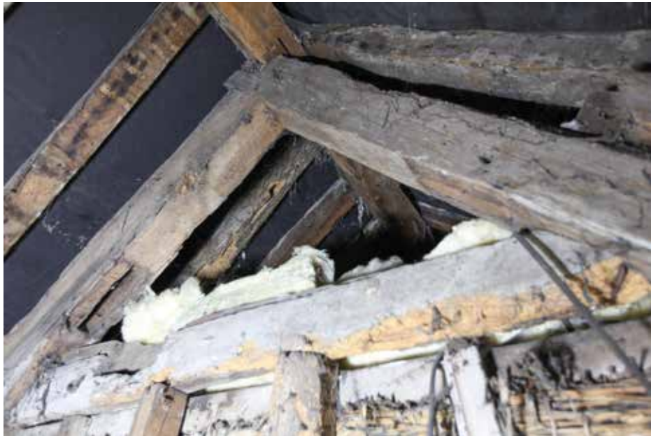
Plate 26 above: Central range Queen strut truss with additional principal rafter; increasing the pitch of the roof and inserted oak studwork to carry reed and plaster for the plastered ceiling below.
