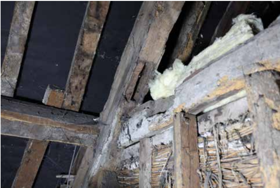
Plate 28 above: Detail of the central range truss showing the mortice in the principal rafter of the earlier raised collar.
