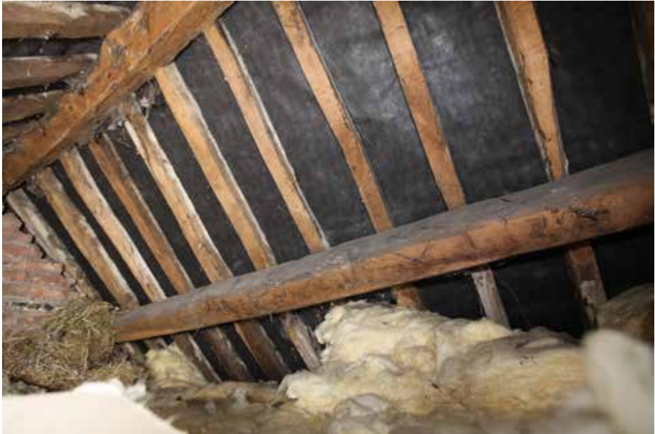
Plate 24 above: Purlin and massive ridge beam to the northern range.
