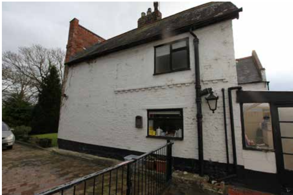
Plate 66 above: Brickwork to dairy wing, with decorative dentilled brick band and original opening to dairy window at ground floor level. Modern window to first floor.
