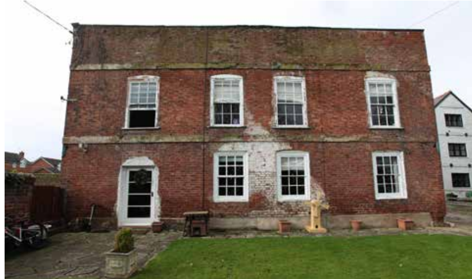
Plate 4 above: The east elevation of ca. 1720-1730 of elegant simplicity and subtle articulation in the form of brick bands was a single unified composition, adopting the principles of the golden section. The protocol for the period was to have an attic storey to provide the correct classical proportions. Here the parapet incorporated faux or blind windows, which completely removed the evidence of the former gable frontage. The recessed openings have been later filled in. We can see from this photograph that the former doorway which was blocked up in the late 20th century (second window from the left) did not sit precisely under the first floor window, the reason being that the existing internal wall to the early hall prevented this. This would not have been as obvious as it is now, being a doorway. At some point the original doorway appears to have had a canopy. The square lintel is modern.
