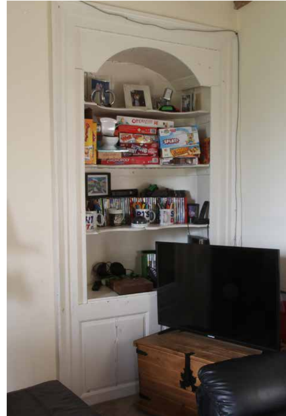
Plate 59 above: Arched china cupboard with stepped architrave, decorative scalloped display shelves, curved back and raised and fielded panelled base, ca. 1730.
