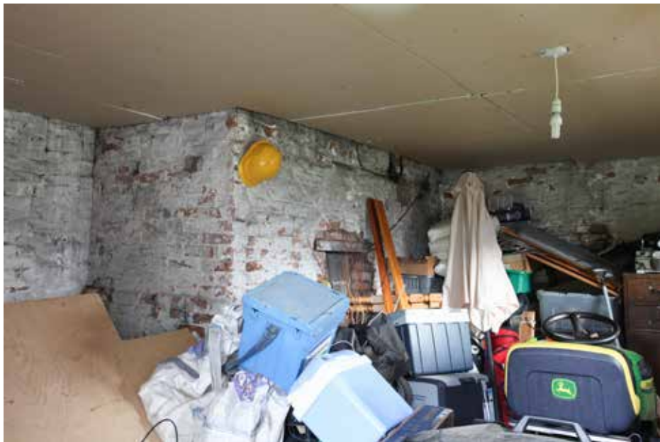
Plate 64 above: Brick masonry for staircase of ca. 1730 inserted into southern wing.
