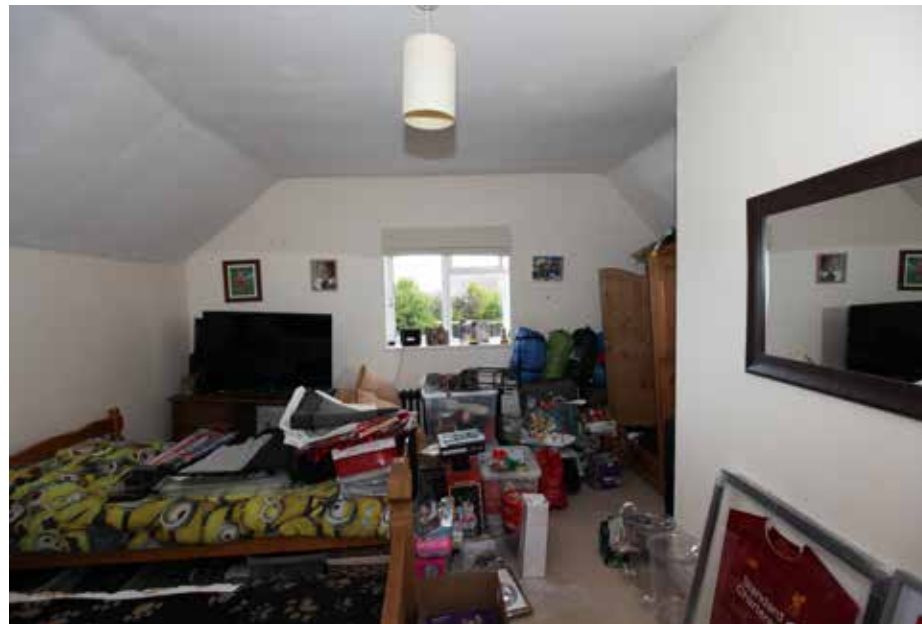
Plate 44 above: Rear bedroom 4, with inserted brick wall to the right, which forms the core of the later inserted staircase. The window on the west wall is a modern replacement.
