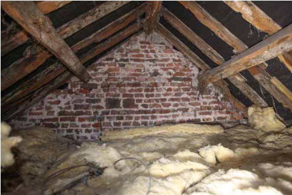
Plate 27 above: Central range - west brick gable with purlins.
