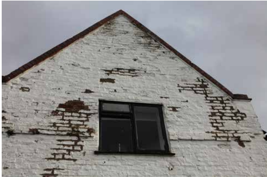
Plate 65 above: Brick gable to west end of southern wing of ca. 1680-1700, with raised brick band and remodelled window.
