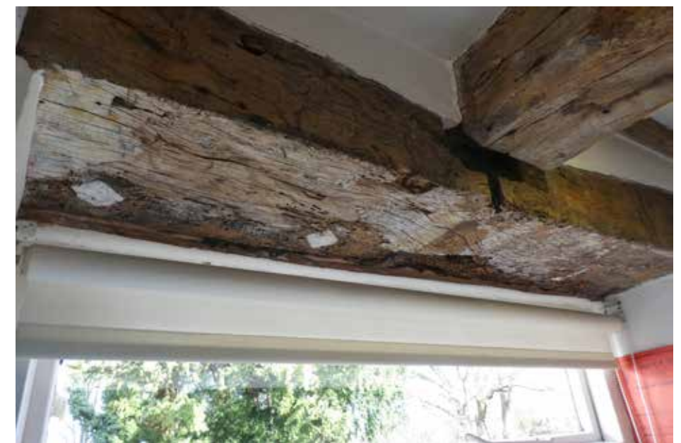
Plate 11: The presence of a diamond mullioned oak window, which would have been unglazed and perhaps shuttered, within the present kitchen, is indicative of a 'dairy'. The evidence for this is in the original oak lintel which incorporates diamond-shaped sockets for the oak 'mullions'. The main spine beam is sitting on this lintel and there are no signs that this is an alteration.
