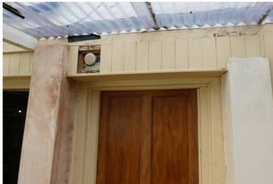
Plate 20 below: Pegged oak door frame (early 18th century) to the original rear door. The inserted door and sub-frame is modern.
