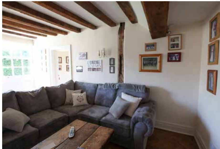
Plate 12: Former Hall, now the Lounge. The joists are of large section with a long span. Also visible is the oak post in the wall and the stop-chamfered transverse beam inserted to support a brick wall above.
