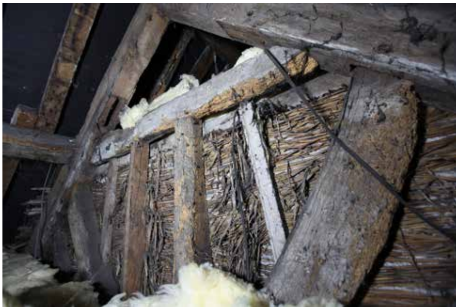
Plate 7: The central truss. The paired curved Queen struts are visible here, as is the timber studwork which incorporates reed and plaster for the raised ceiling in Bedroom 2. The mortices for an earlier, higher, collar reveal that the rafters may have been once under-drawn with reed and plaster, suggesting that the truss predates the east elevation.
