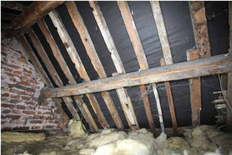
Plate 30 above: Central range purlin and rafters.
