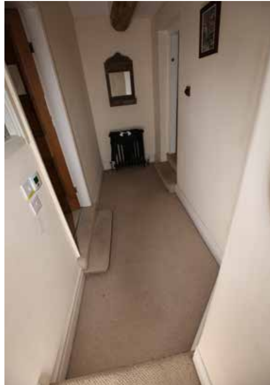
Plate 43 left: Step down to the landing over the former dairy. The floor then steps up into Bedroom 3, part of the c.1730 remodelling.
