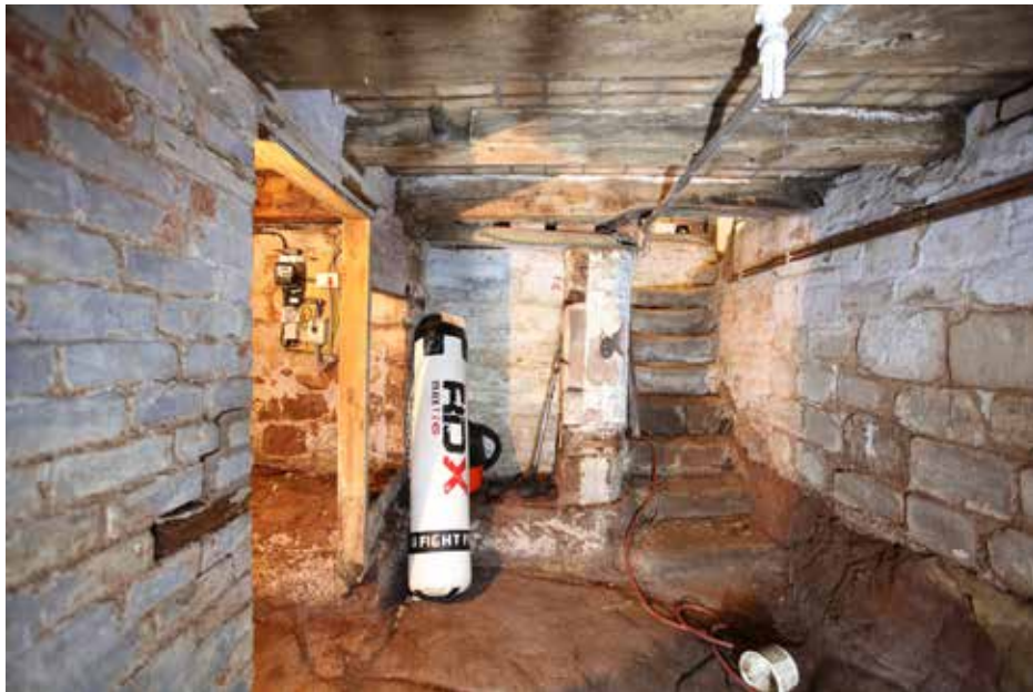
Plate 14: The cellar dates from ca. 1680-1700. The entrance was modified ca. 1730 in order to get access from the staircase hall. The original access to the cellar may have been central (see panel of brickwork to the left of the stone pier). Note the massive oak joists, which are re-used parts of a timber-framed building.
