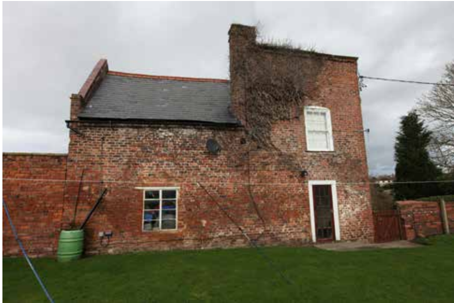
Plate 63 above: Southern wing of c. 1680-1700, with raised parapet, remodelled stack and inserted sash window to east.
