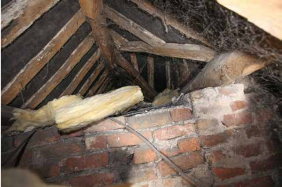
Plate 22 above: 18th century brickwork of two phases to the northern range. The raked valley rafters visible relate to the brick chimney.
