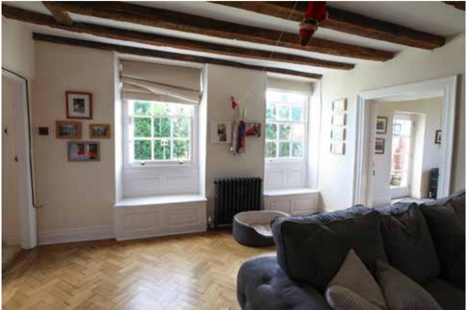
Plate 53 above: Hall with panelled lined windows of c.1730, that to the right has been relocated here from the adjoining parlour. Plate 54 below: oak post of timber frame with pegged joints for horizontal rails.
