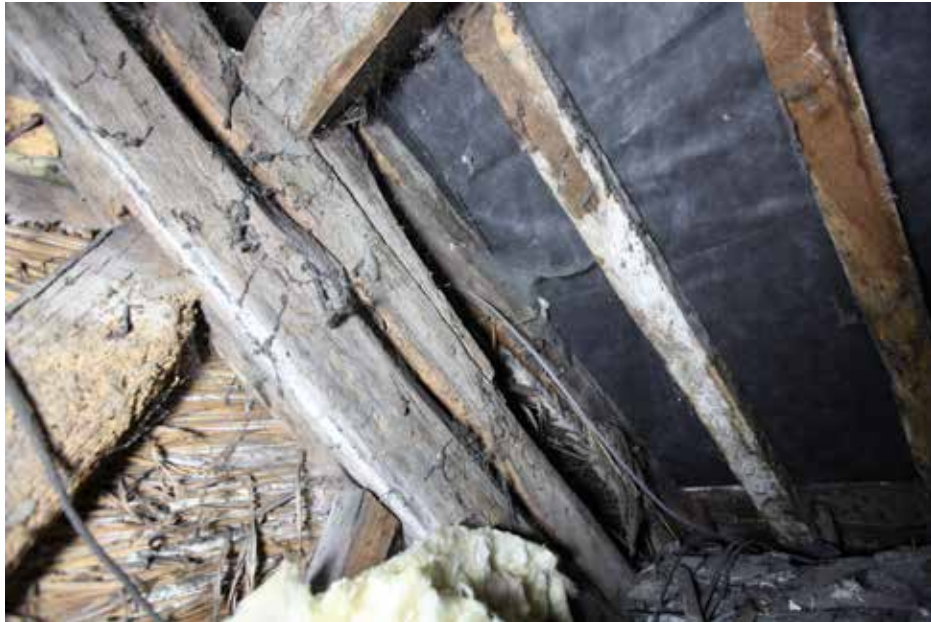
Plate 25 above: central range Queen strut truss with secondary principal rafter.
