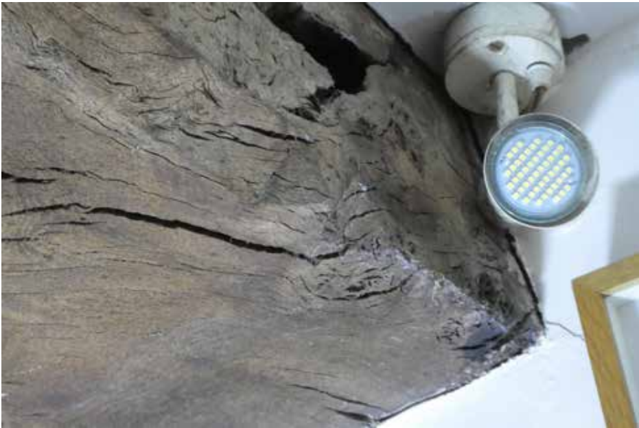
Plate 55 below: Detail of oak chamfered beam.
