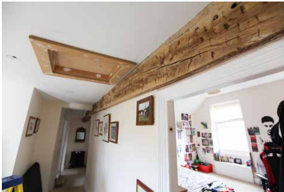
Plate 8: The oak beam which spans the central and northern ranges supports the two trusses. The pegged joints can be seen over this doorway.
