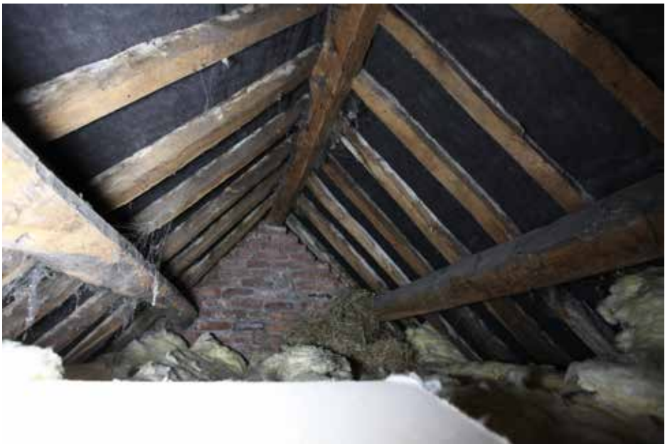
Plate 23 above: West brick gable to the northern range, with purlins.
