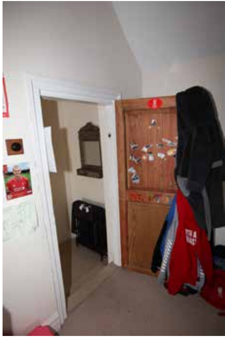
Plate 40 above: 2-panel C18 door to bedroom 3, ex-situ. The frame is 18th century.
