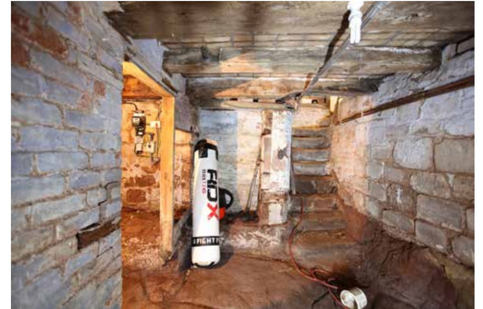
Plate 60 above and Plate 61 below: Cellar with stone masonry of ca. 1680, re-used joists (probably 16th century)
