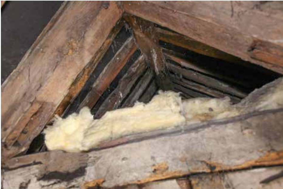
Plate 29 above: central range roof to the east showing the ridge beam and rafters
