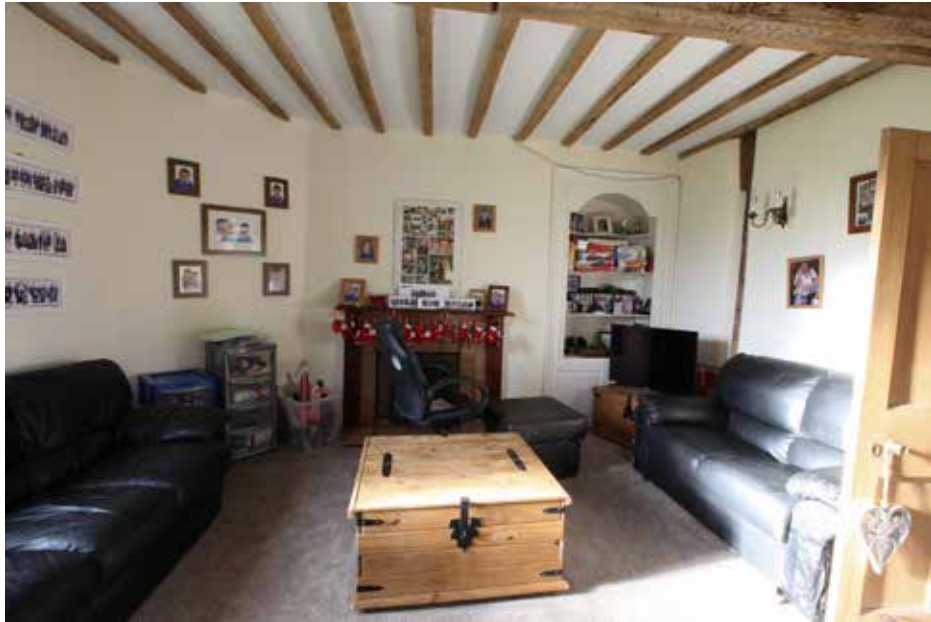
Plate 56 above: View of the parlour, with corner fireplace to the left (blocked-up), later fireplace to the centre and arched cupboard of c.1730 to the right.
