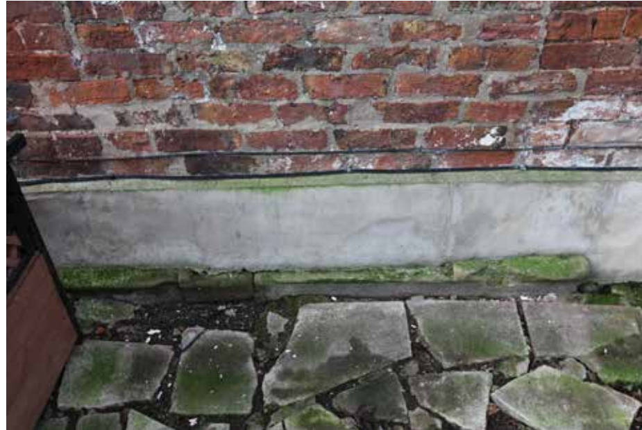
Plate 19 above: Stone moulded doorstep threshold and straight joints to the original front door.
