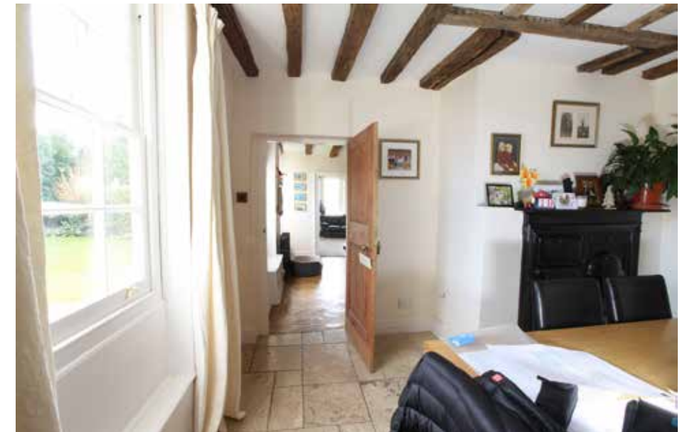
Plate 46 above: Dining Room, looking into the Lounge. 2-panel 18th century door, probably ex-situ, and remodelled ceiling joists.
