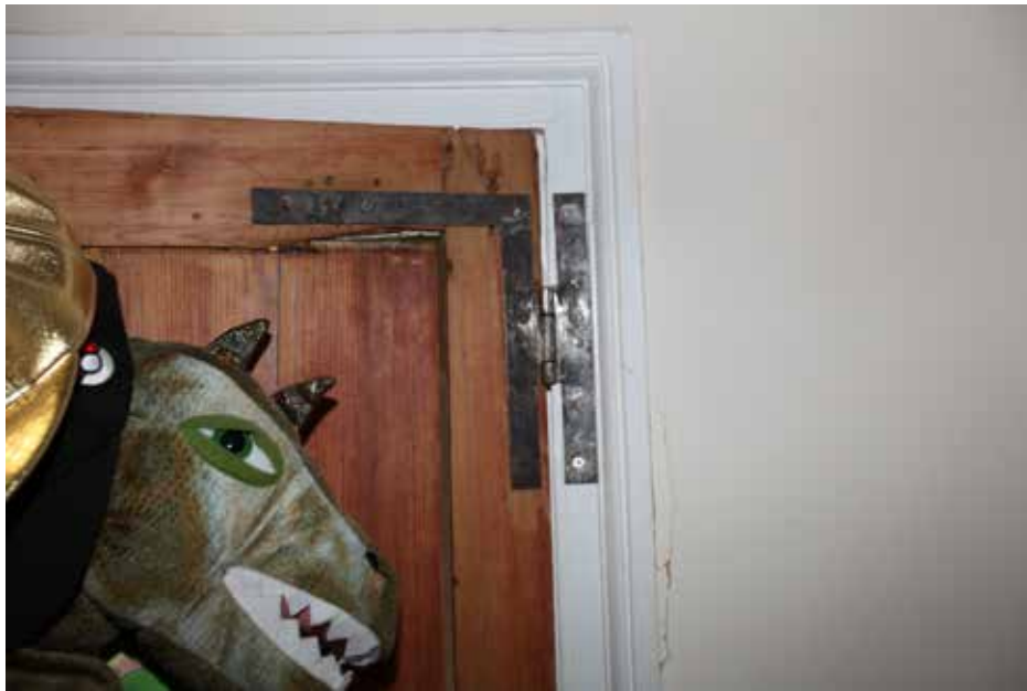
Plate 42 above: HL hinges have been screwed onto all of the 2-panel doors at first floor level. These are ex-situ but re-used 18th century hinges.
