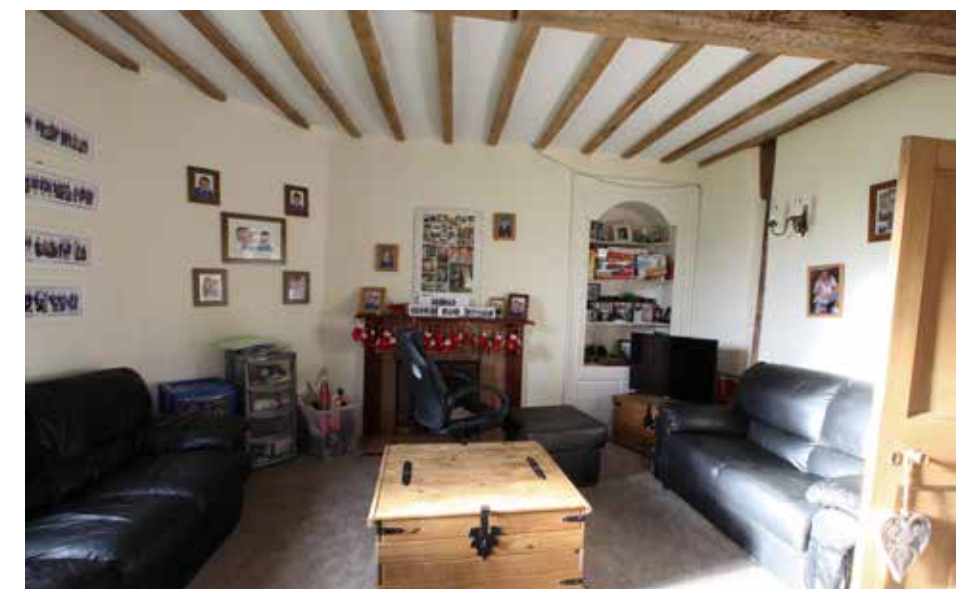
Plate 13: Parlour with brick angle for the corner fireplace to the left, a later hearth to the centre, with modern surround, and an arched corner cupboard to the right of ca. 1730, for displaying best china. The ceiling was originally underdrawn with plaster.
