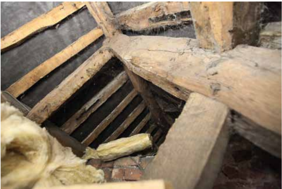
Plate 21 above: Queen strut truss to the northern range.
