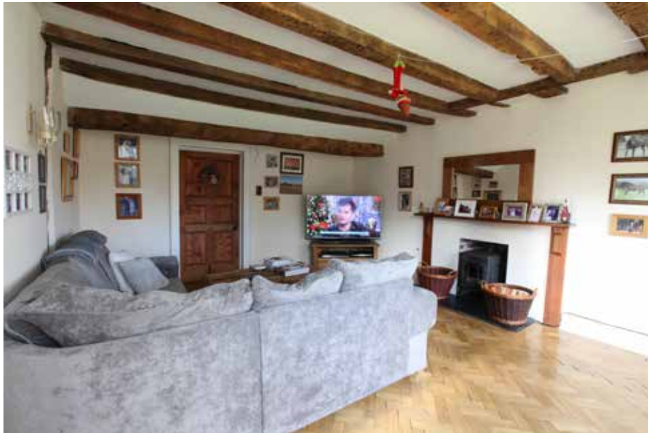
Plate 49 above: View of former hall, with early joists, modern fireplace and trimmed joists around former chimney breast.
