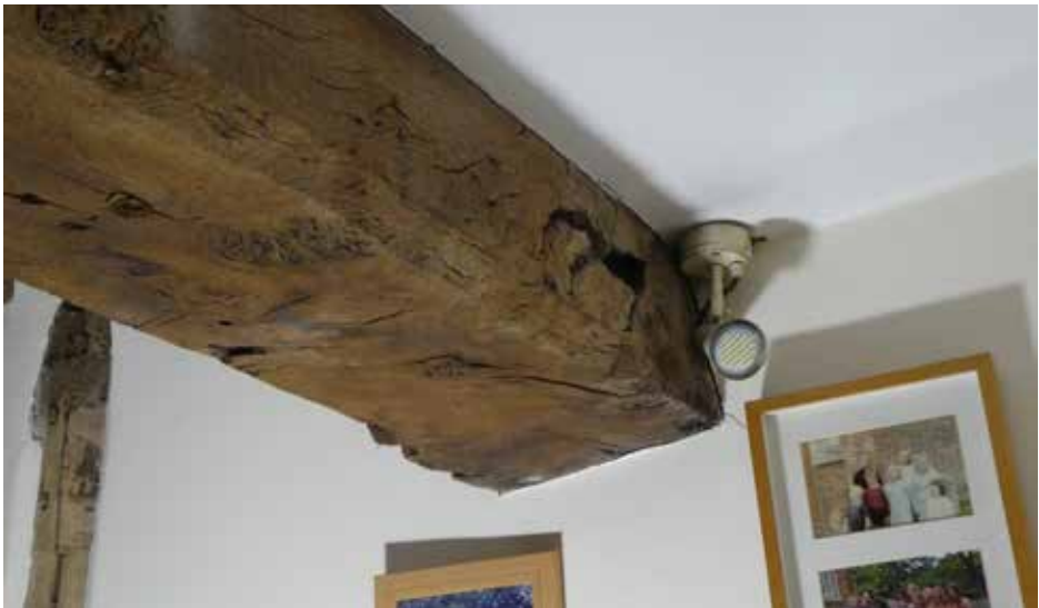
Plate 55 below: Detail of oak chamfered beam.
