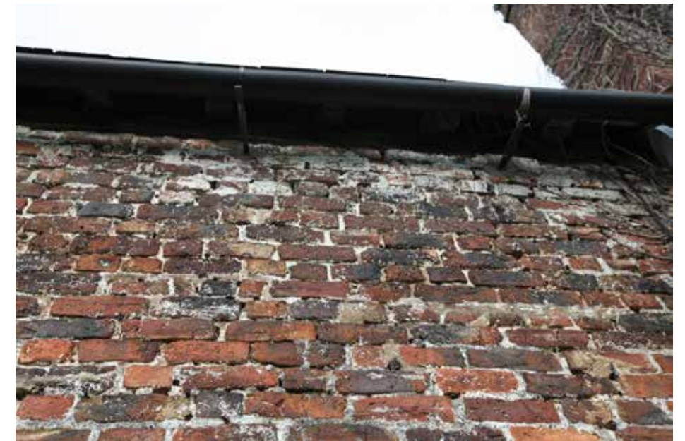
Plate 15 above: Brickwork of ca. 1680-1700, formerly limewashed.
