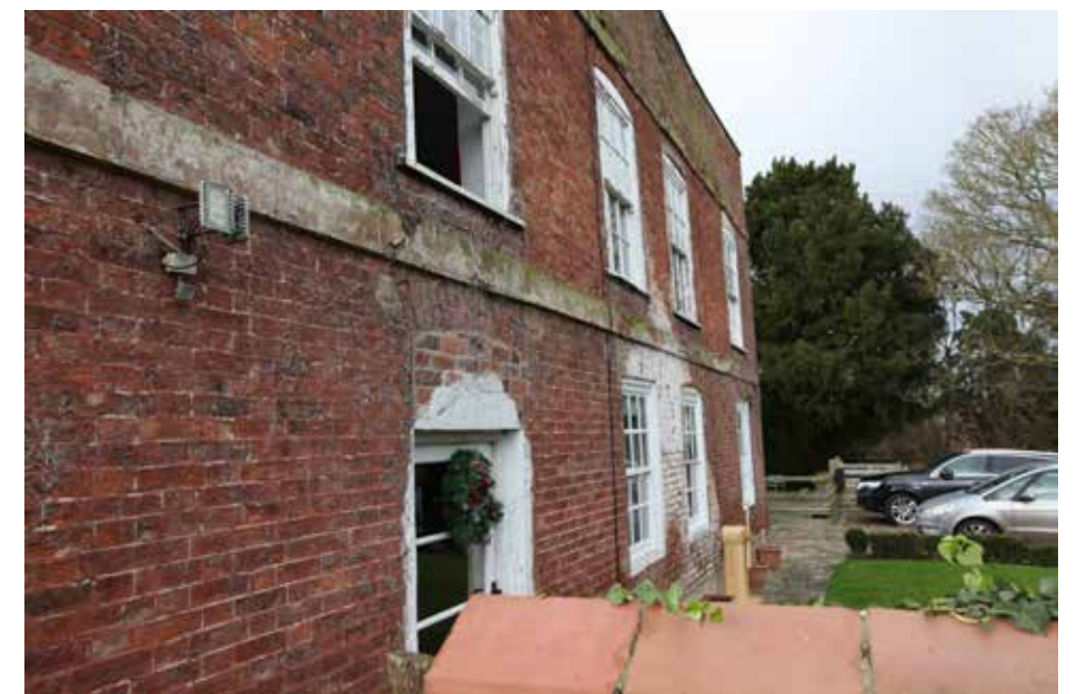
Plate 16 above: Brickwork of the late 17th century to the 'dairy', with dentilled band Plate 17 below: Flemish bond brickwork with 'tuck pointing' of lime putty of ca. 1730.
