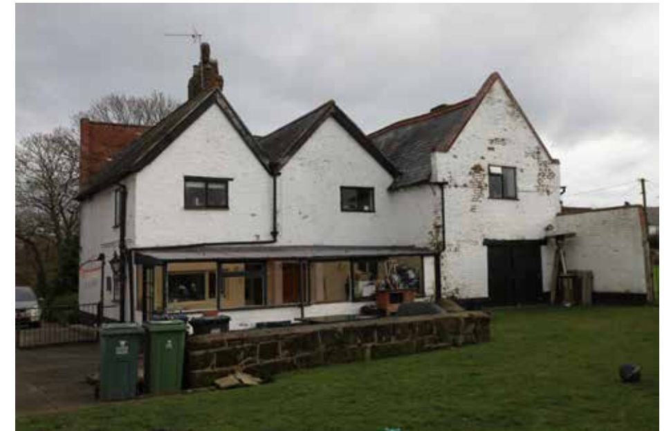
Plate 6 above: The west elevation incorporates a slightly taller wing to the south, with raised coped gable, of ca. 1690-1700 and a pair of gables to the centre and north which are coeval. These roofs were probably built immediately after the south wing.
