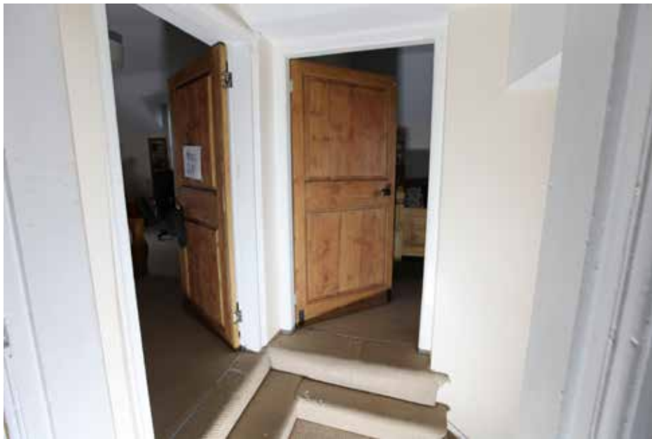
Plate 18 above: Inserted 18th century doors within original 18th century openings at the head of the staircase. The doorway to the right has a stop-chamfered frame.
