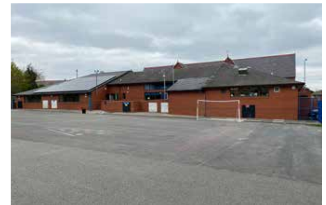
View of the Southern elevation across the playground which will be the location of the proposed new extension
