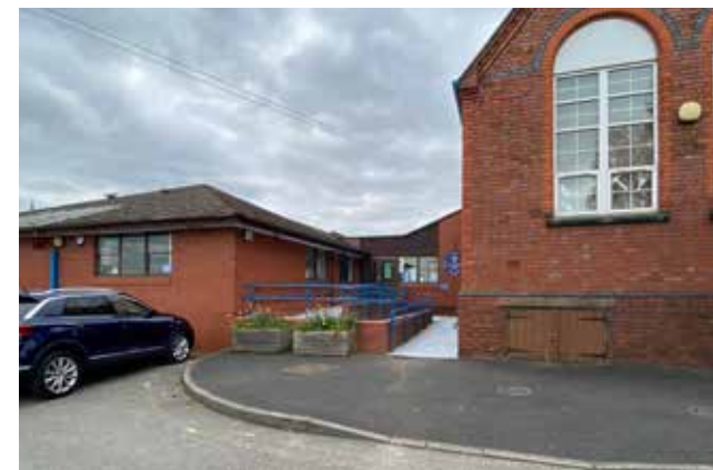
View of the existing building entrance which forms the connection between the original school building and the 1985 extension
