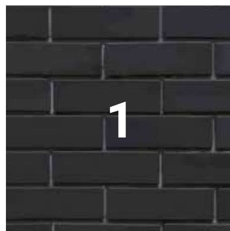
Grey/Black Brick Stretcher Bond | Dark Grey Mortar
