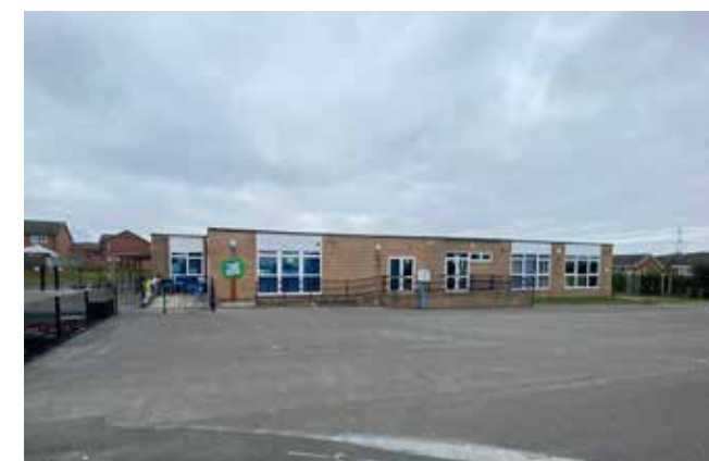
View towards the side elevation across the playground
