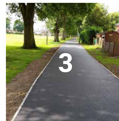
Asphalt concrete surfacing
