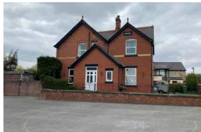
View of the Front elevation from the school playground illustrating the interesting roof scape
