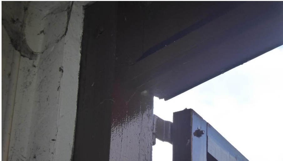
Figure 4.13. Area above garage door where bat fell from
