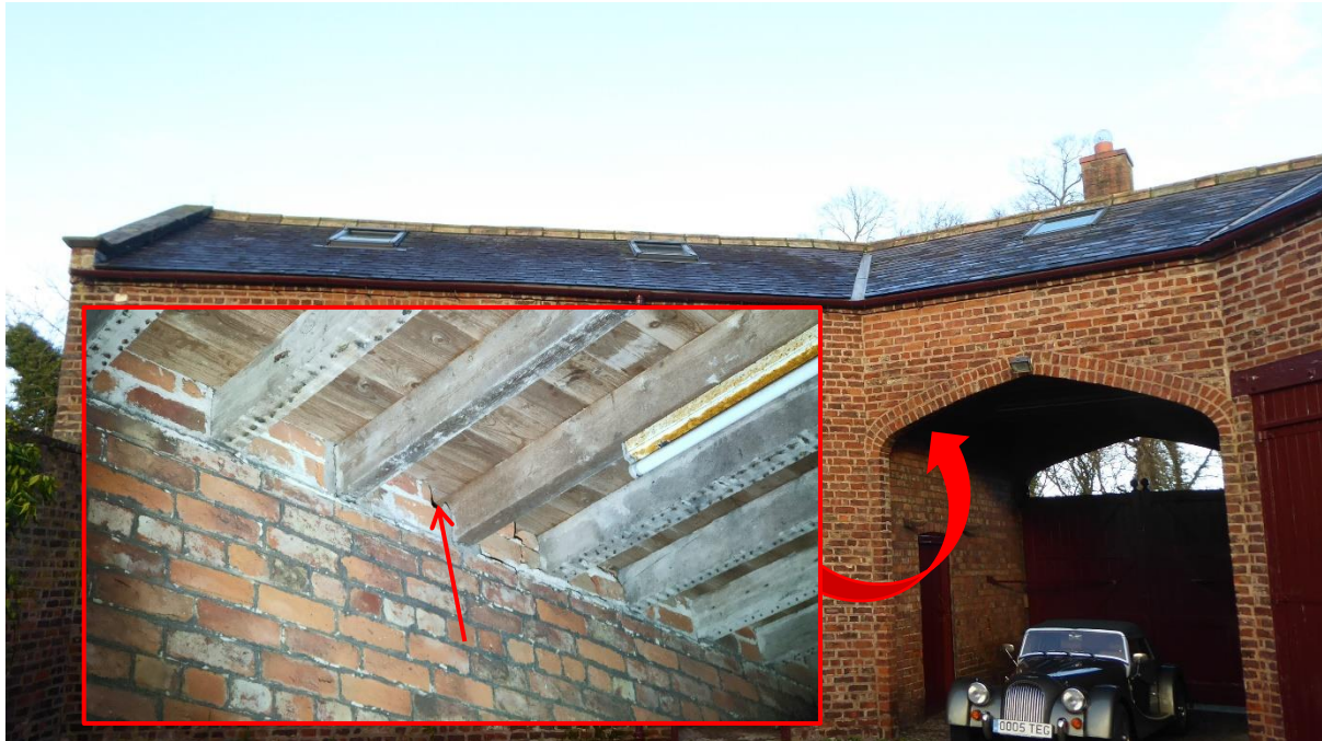
Figure 4.15. BLE roost entry point
