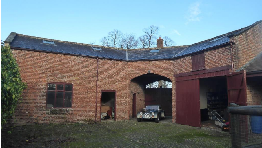
Figure 4.3. External view of stables from south
