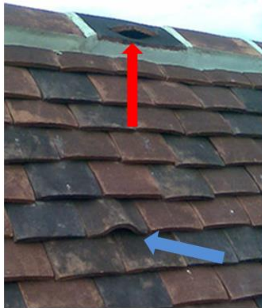
Figure 6.3. Example ridge and access tiles
