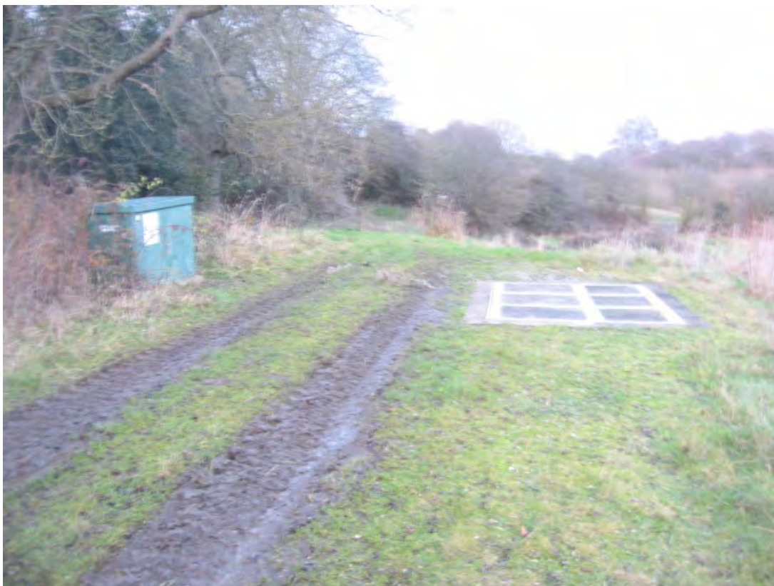
Photo 5 – Underground tanks relating Welsh Water
