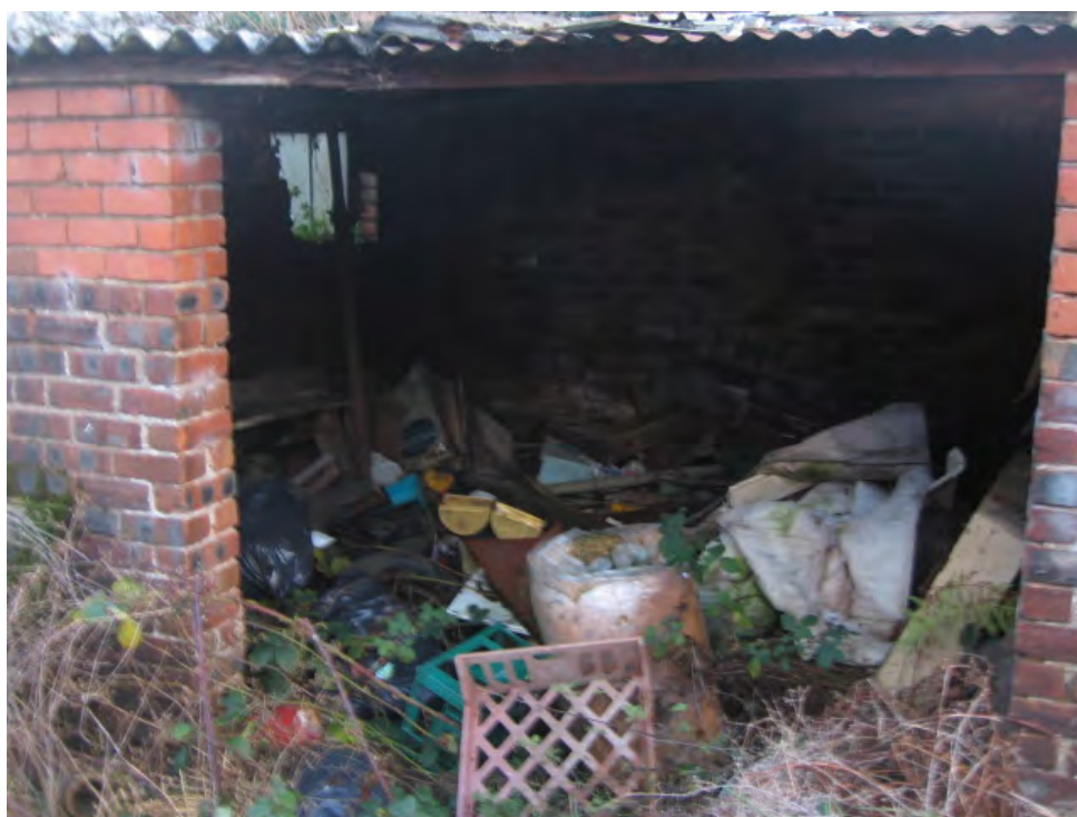
Photo 2 – View of contents of farm buildings with general waste
