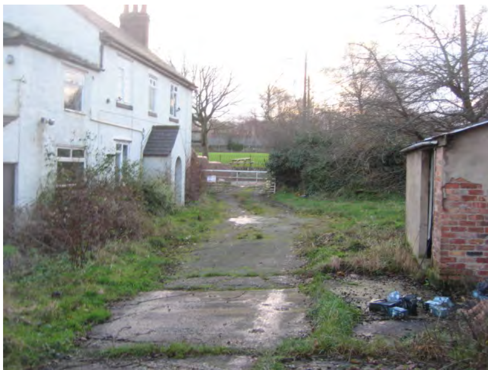
Photo 1 –General view south west of the farm building and the access from Dodds Lane
