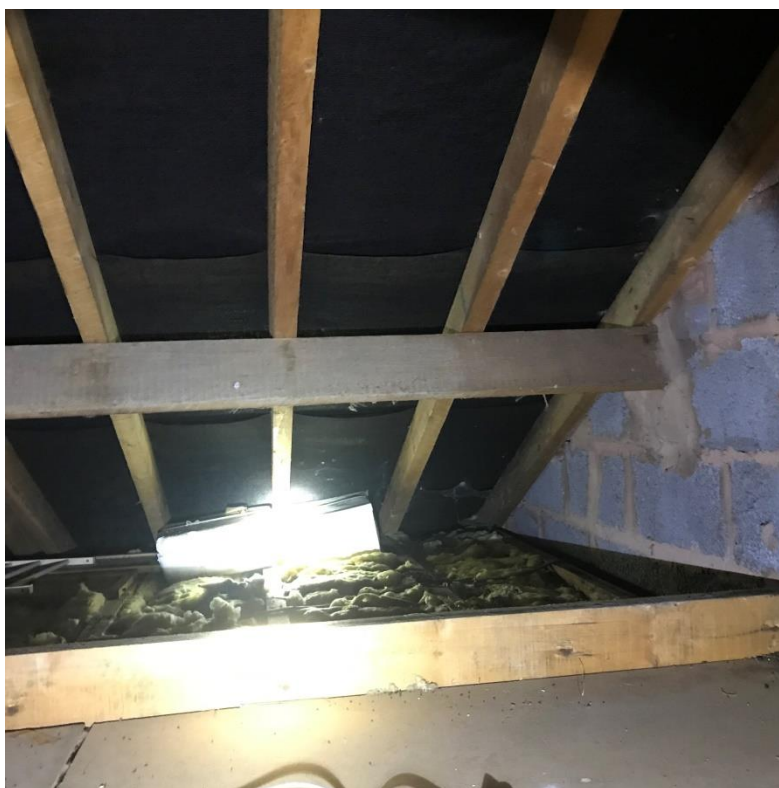
Plate 10 – Character of the loft space
