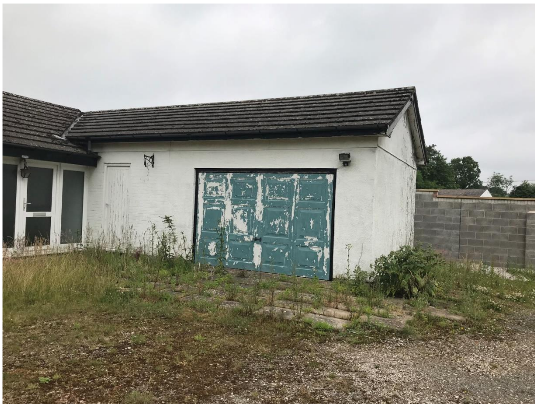
Plate 3 – A view of the east facing wing
