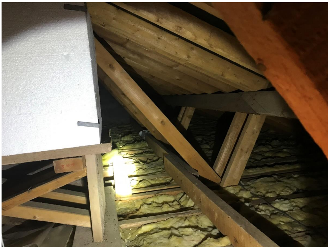
Plate 11 – Character of the loft space
