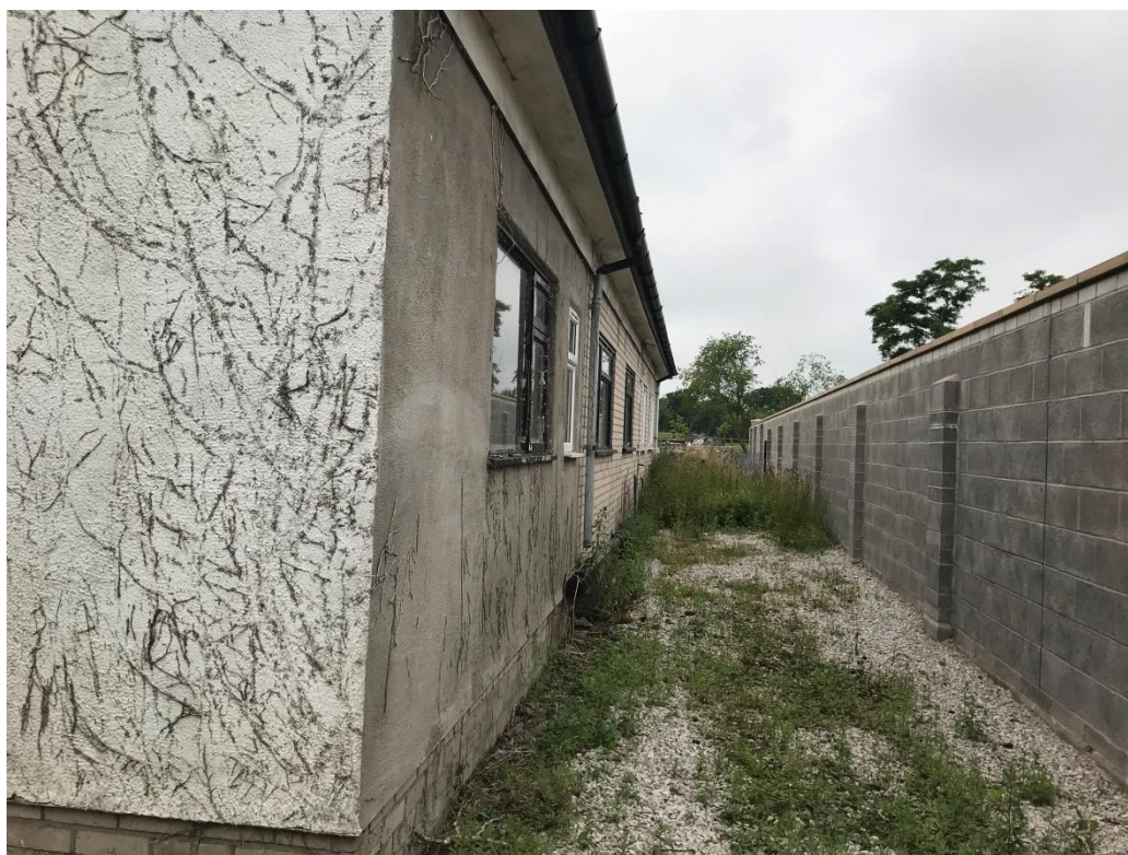
Plate 4 – Rear of the dwelling
