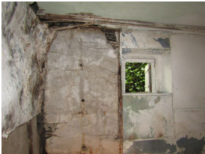
Photo 2: LHS bats emerged from the open window in ground floor room near Northwest corner of the building.
