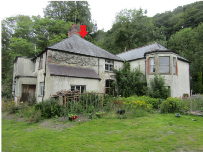
Photo 1: Soprano Pipistrelle (red arrow) bat roost access point.
