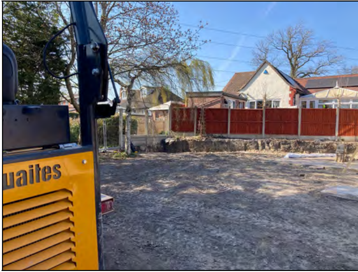
Plate 1 – Ground in lawn area prior to barrier layer placement
