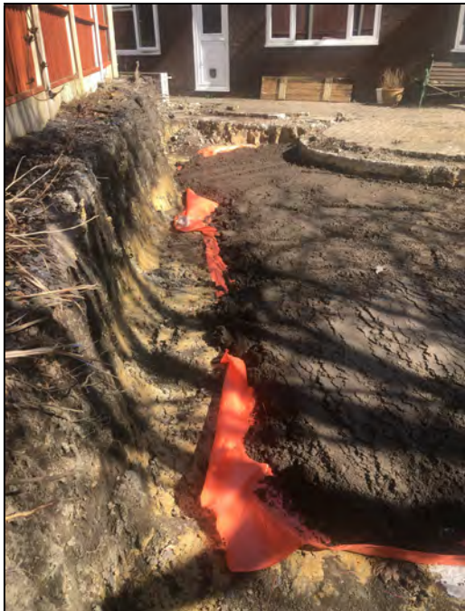
Plate 2 – Warning layer and soil placement
