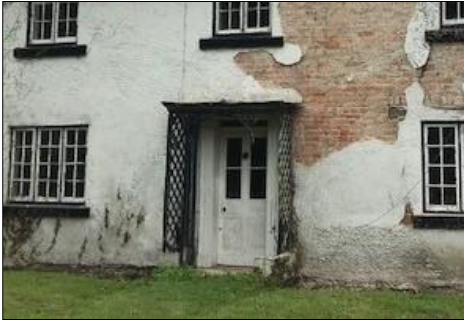
Photograph 1 showing the porch
