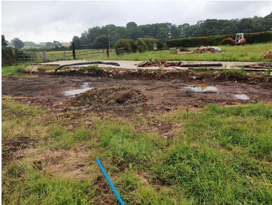
Figure 4.3. Bare earth and hardstanding
